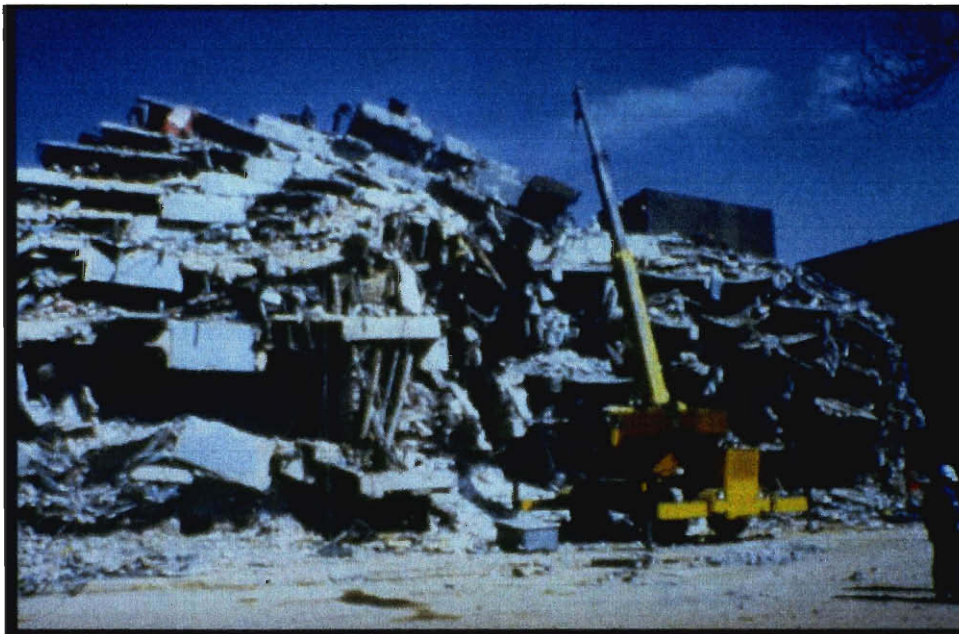
Figure 2.6: Hospital Collapse in Mexico City due to Resonance (1985) Source: NGDC (2001)
