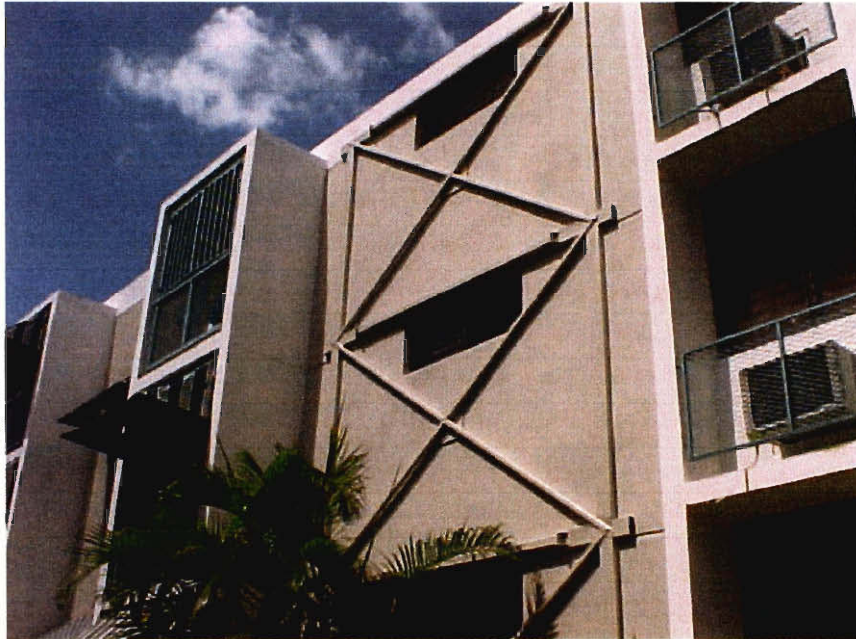
Figure 2.7: Steel Bracing of Structure in Puerto Rico Photo taken by CSA Project Team (2001)
