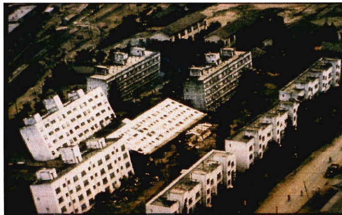
Figure 2.5: Soil Liquefaction Results in Niigata, Japan Source: NGDC (2001b)
