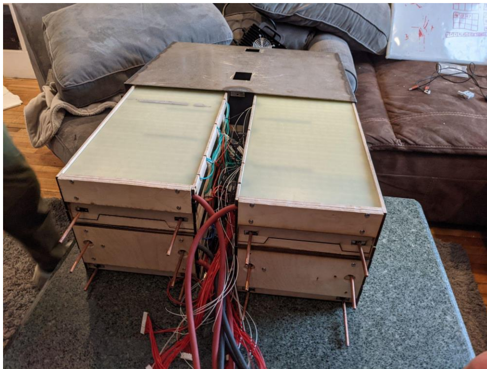
Figure 64. Initial fitment tests of the battery stacks in the battery box.
