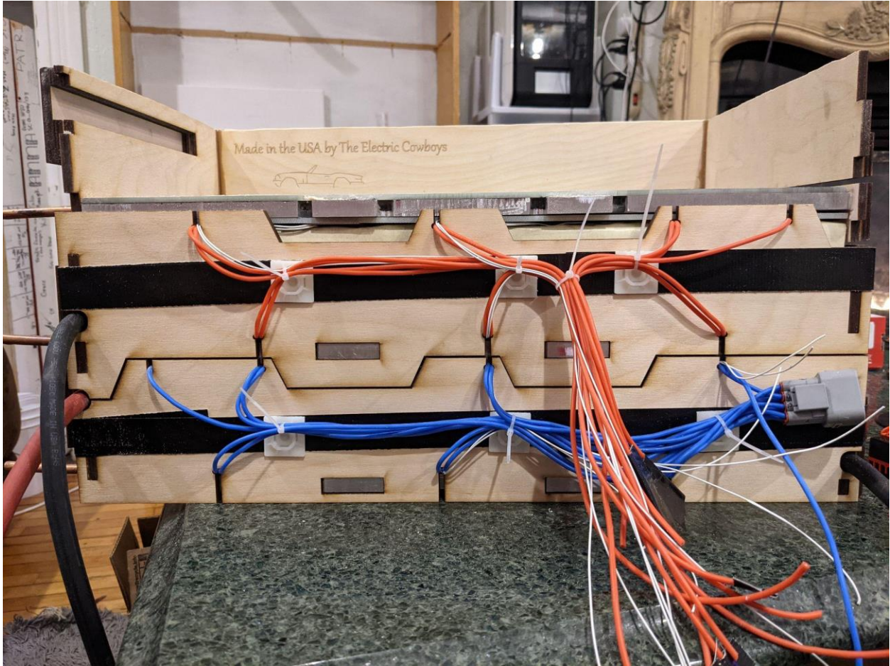
Figure 40. Mid way through final assembly of the battery modules
