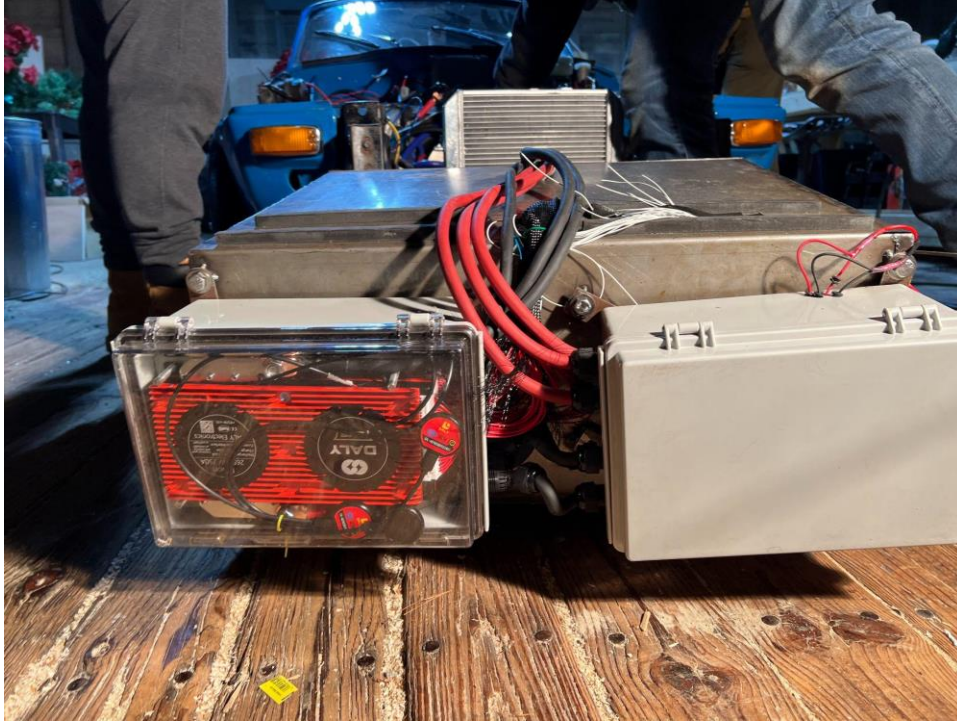
Figure 67. Finalized Integration of Junction Boxes 1 & 2 onto the Accumulator Housing
