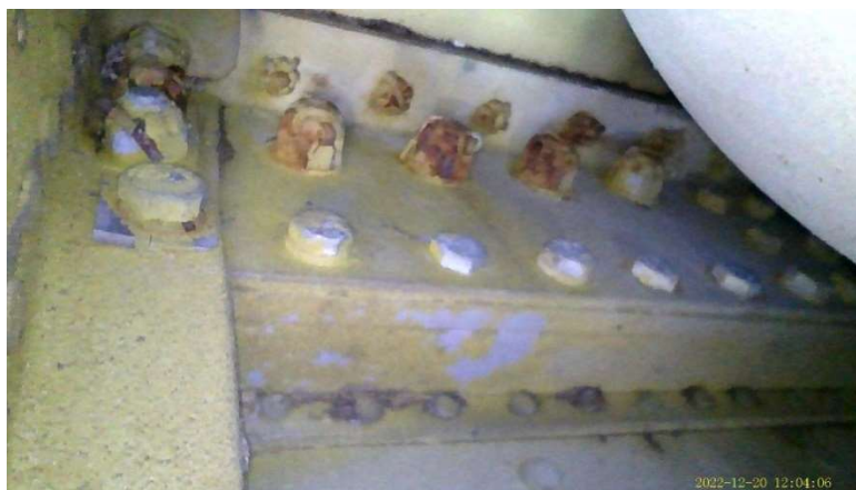
Figure 11: Metal Box Structure Encasing End of Bracket D
