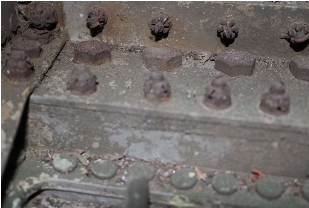
Figure 23: The above image was taken by the team of the internal wing structure using the NTS300 endoscope.
