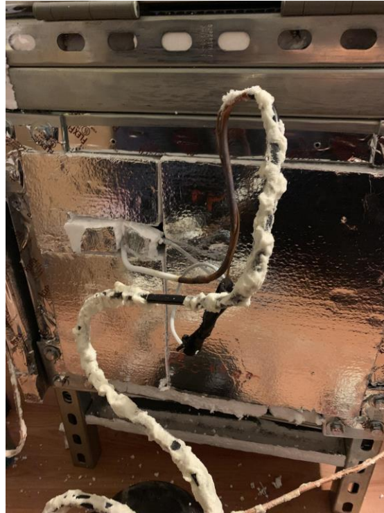
Figure A.6: The compressor unit being fitted on and installed into the unit.
