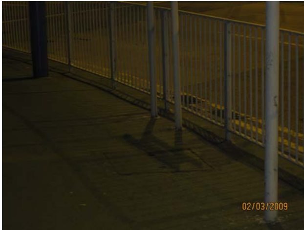
Picture K-3: Sign Post Obstruction
