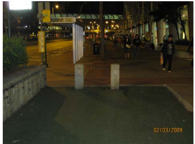
Picture K-18: No Road Surface Markings
