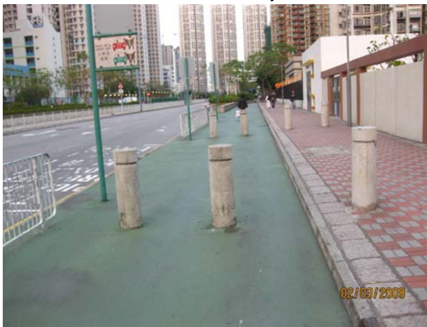
Picture K-9: Unnecessary Bollard
