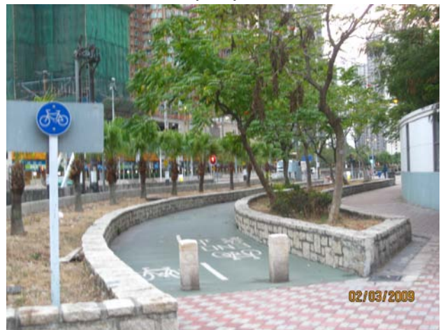
Picture K-16: No division sign for pedestrian walkway/bicycle track
