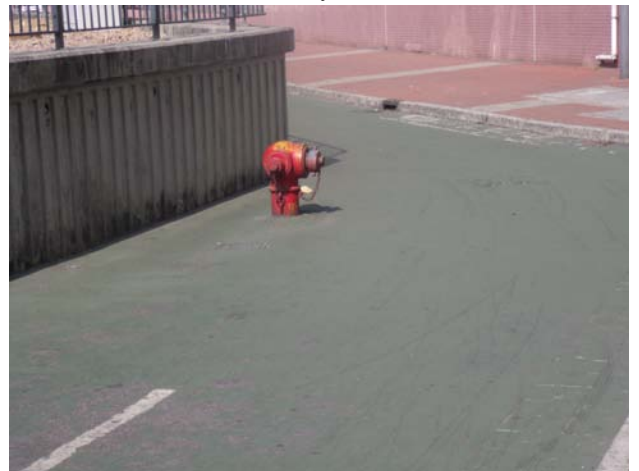
Picture K-6: Fire Hydrant Obstruction
