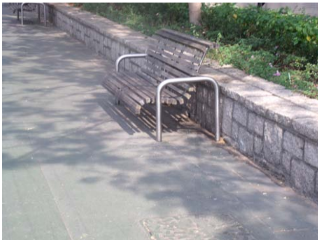
Picture K-5: Bench Obstruction
