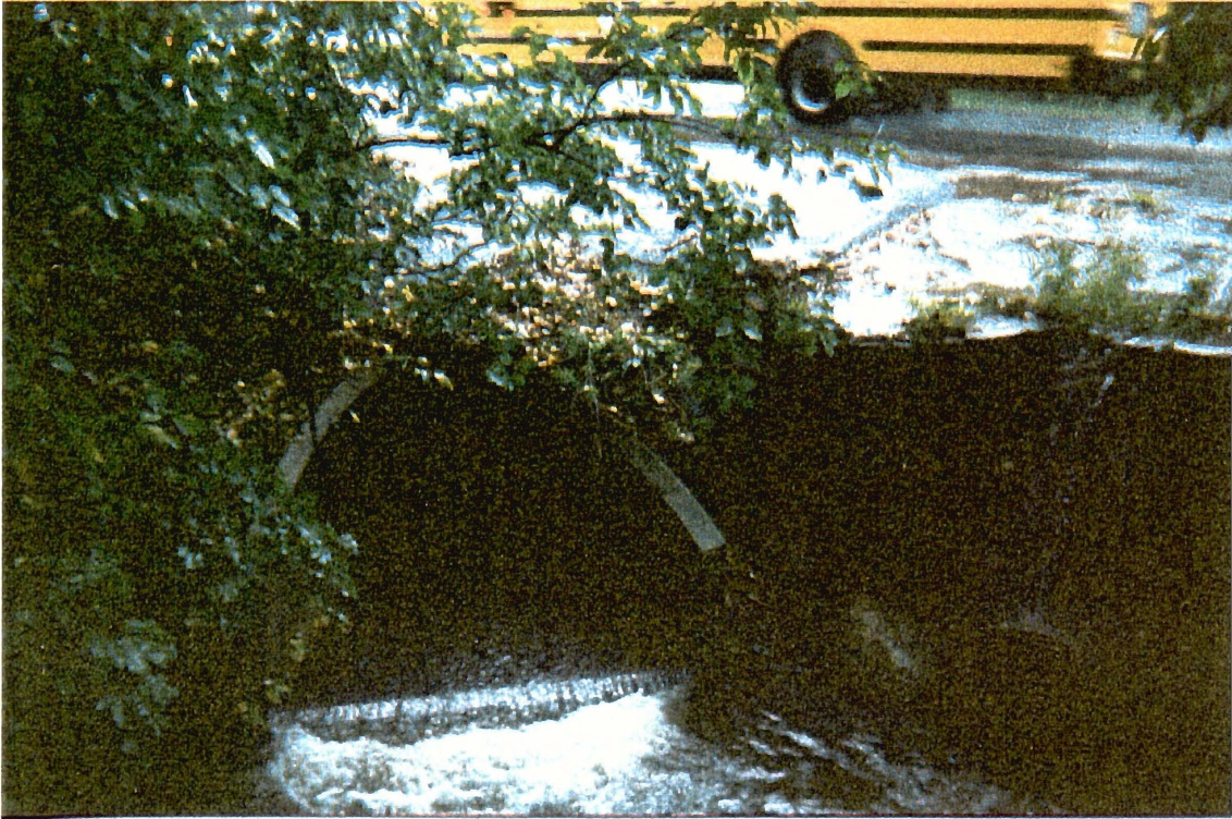
FIGURE 5: HIGH VELOCITY OF WATER COMING DOWN ARARAT STREET. AT A HIGH VELOCITY, THE EROSION OF THE ROAD SHOULDER AND STREET SAND IS EXTREMELY LIKELY.
