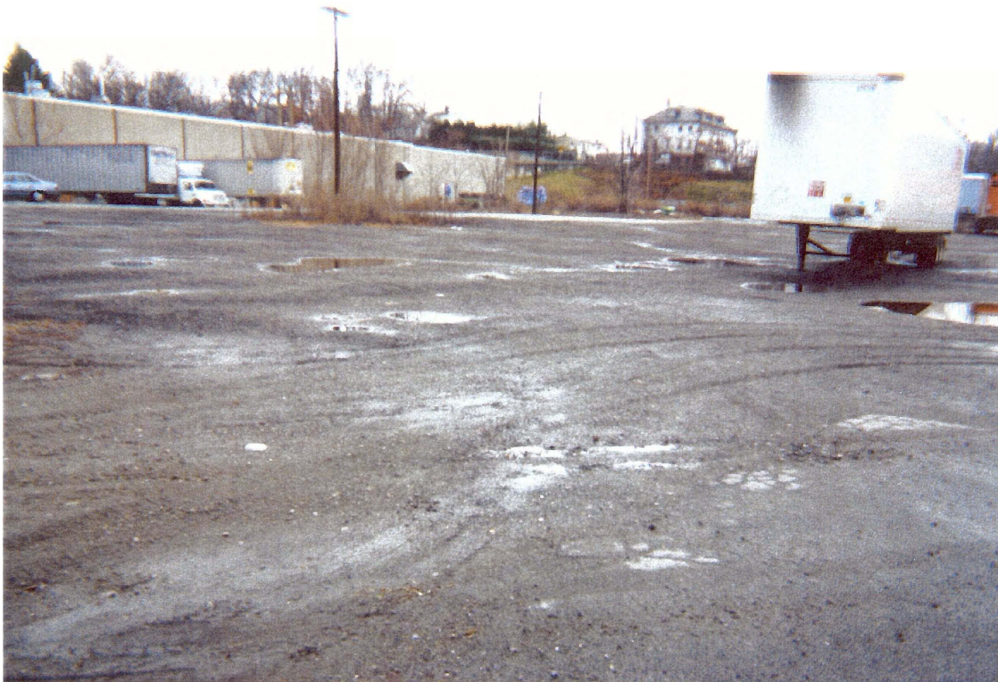
FIGURE 13: UNPAVED PARKING LOT ON PULLMAN STREET. DURING A HEAVY RAIN, THE PARKING LOT MAY DRAIN INTO A CATCH BASIN IN THE STREET.
