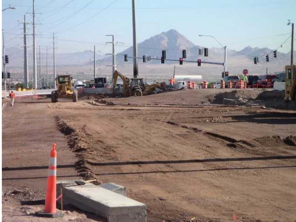
Figure 1: Subgrade Source: Nevada Department of Transportation
