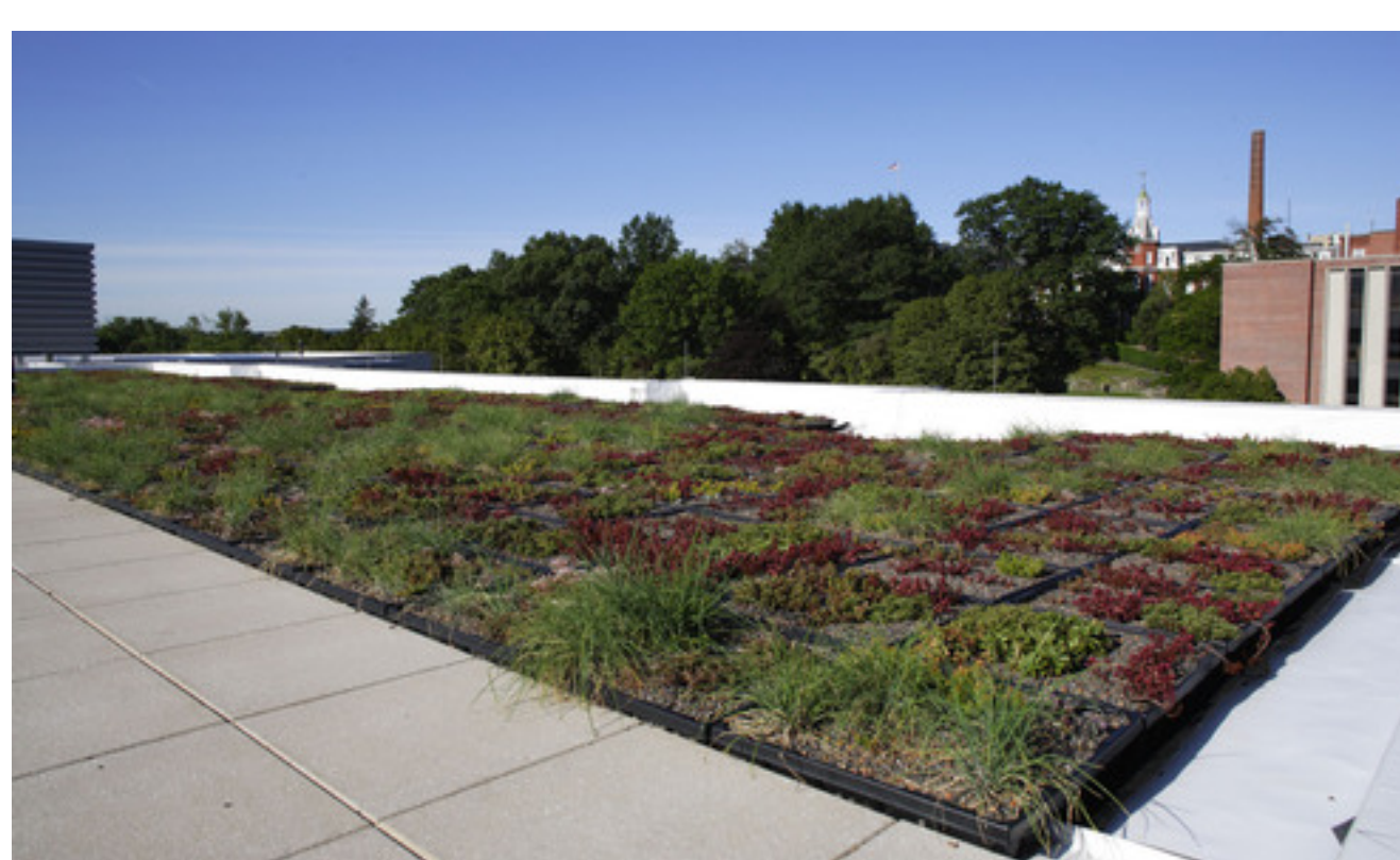
East Hall, Worcester's first green roof
