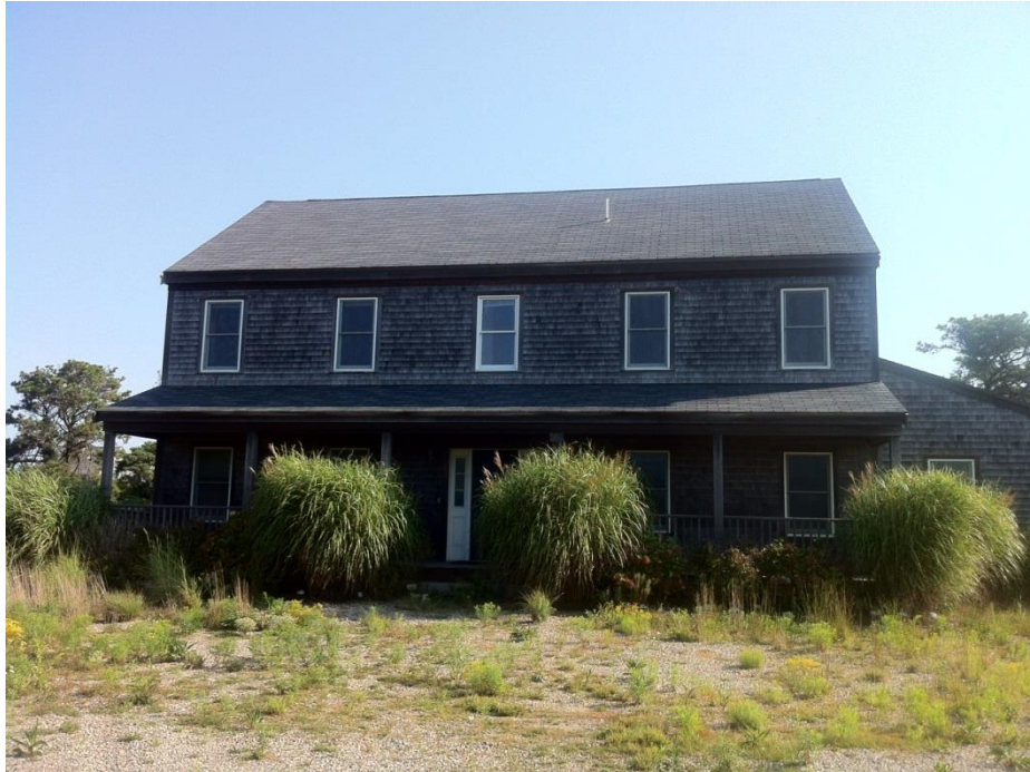
Figure : Clifford House Front View (NHA Properties Inc.)
