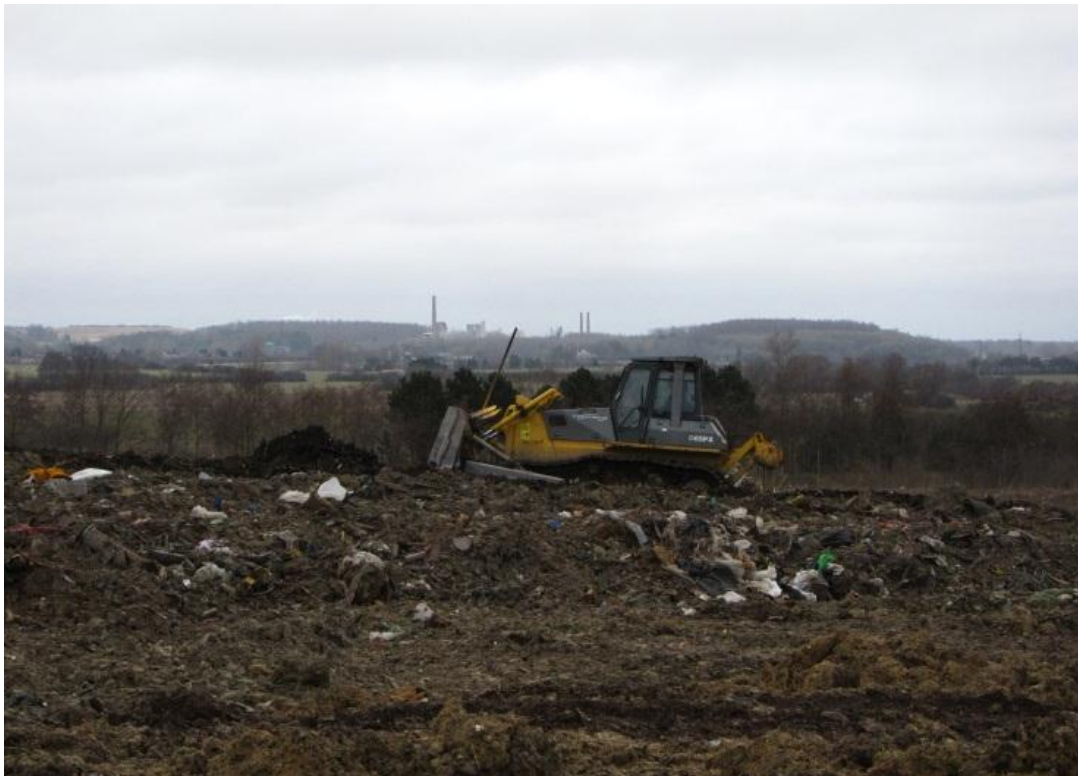
Figure 12: Bulldozer spreading and compacting soil layer to landfill in aftercare
