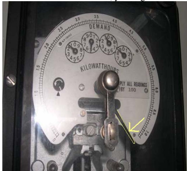
Figure 12: Olin Hall's meter (needle is off the scale)
