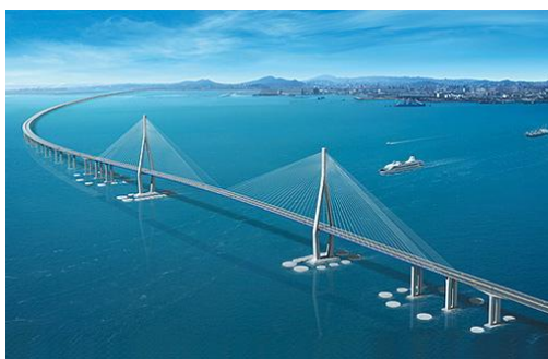
Figure 3. Bridge with 7.5 mile connecting Incheon International Airport
