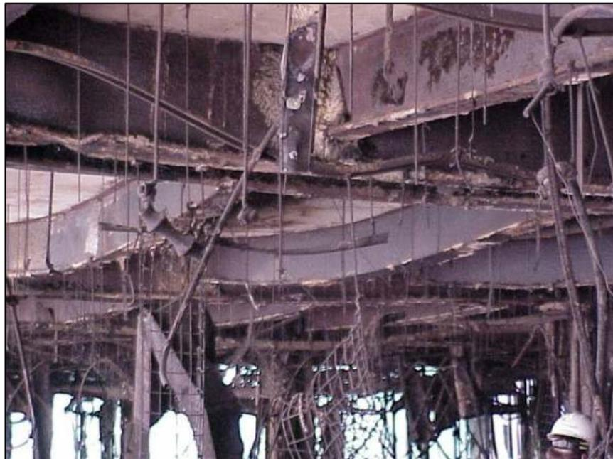
**Figure 22: Deformed Beams in WTC 5 (9<sup>th</sup> Floor) (View 2)**
