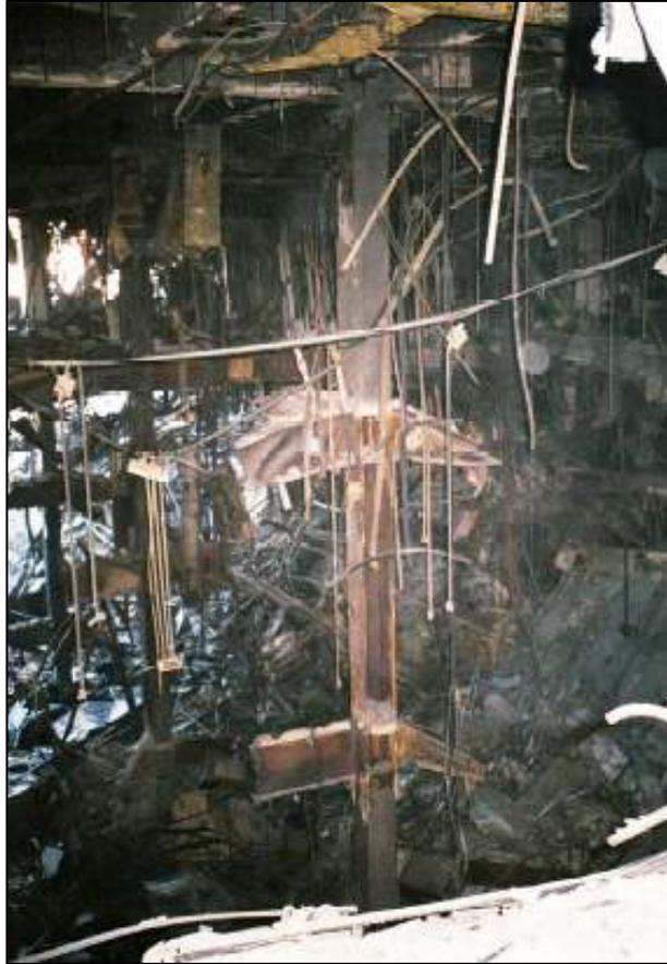
**Figure 26: Localized Structural Collapse of WTC 5 (Perspective 4)**
