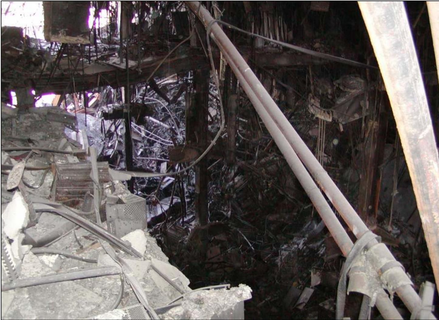
**Figure 25: Localized Structural Collapse of WTC 5 (Perspective 3)**
