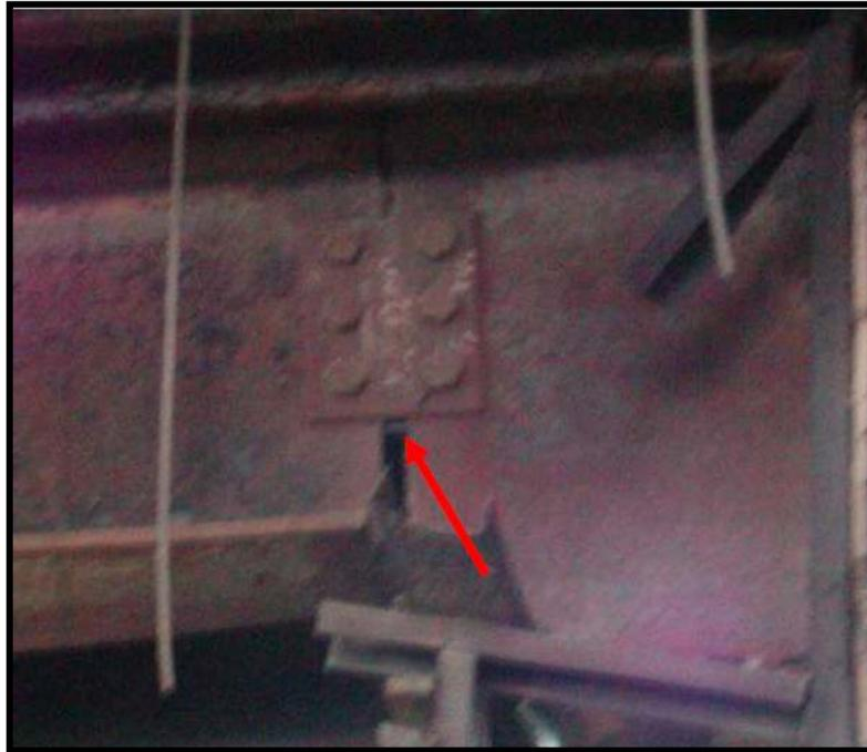
**Figure 121: Photograph of the Shear Tab Connection (WTC 5) (NIST)**
