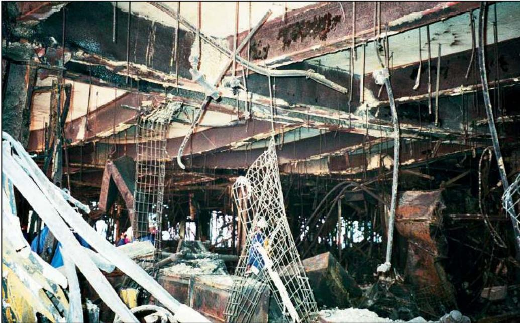
**Figure 21: Deformed Beams in WTC 5 (9<sup>th</sup> Floor) (View 1)**
