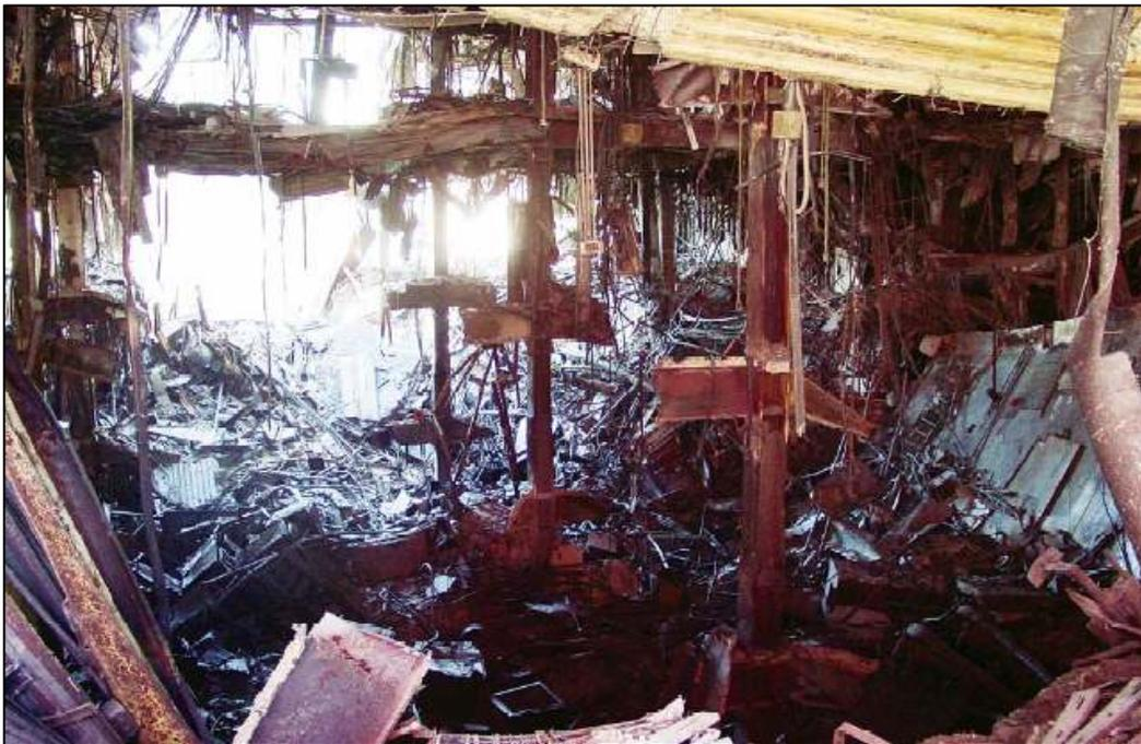
**Figure 24: Localized Structural Collapse of WTC 5 (Perspective 2)**
