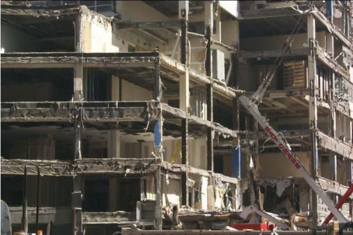
**Figure 34: Exterior View of WTC 5 (Shielded Columns)**
