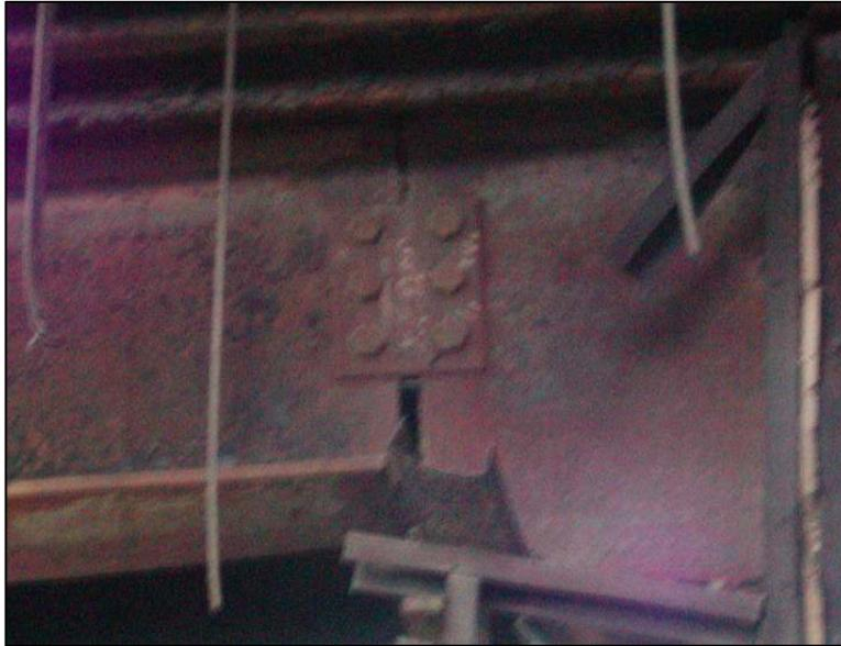
**Figure 28: Typical Shear Connection in WTC 5**
