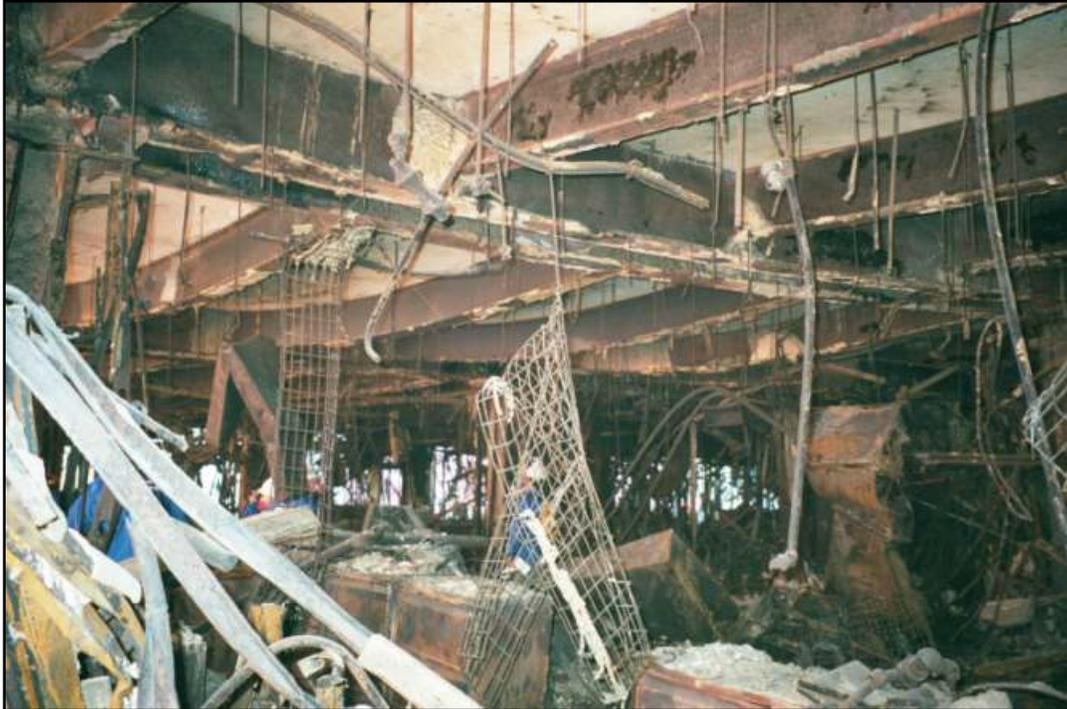
**Figure 5: 9<sup>th</sup> Floor of WTC 5 After Fire Burnout**
