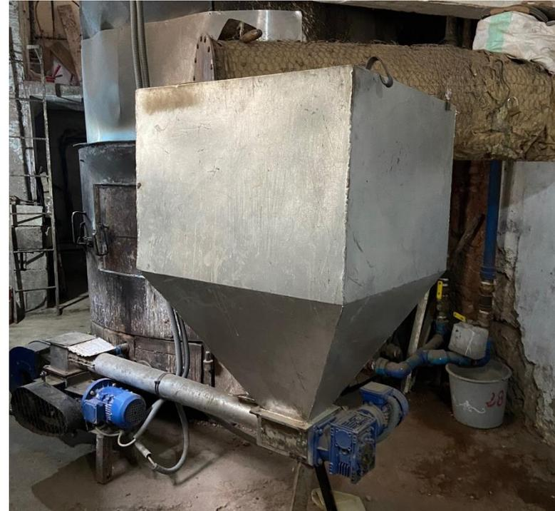
aspects of a modern heating system, providing enormous economic and energy savings. This is because a feeding system eliminates all ambient heat loss that occurs when opening the boiler door to add fuel. Furthermore, by concentrating added fuel to the center of the fire, it makes sure the fuel is burned to completion further reducing emissions. Based on our data analysis, the feeding system increases the overall efficiency of
