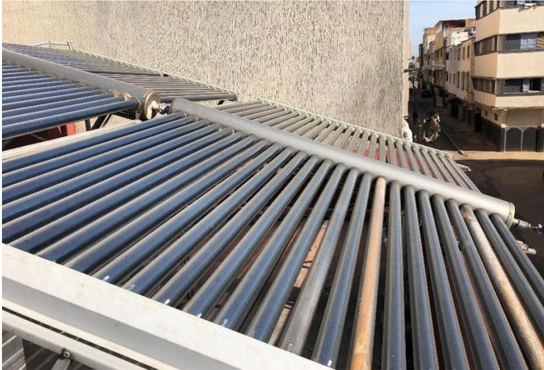
Unfortunately, a solar heating array is difficult to install and maintain due to the current lack of skilled labor specific to sustainable mechanical systems in Morocco. The solar heating array referenced broke in the winter of 2018 due to rust buildup in the water pipes, and since then, the Hammam owner has not been able to find someone to fix the system, leaving it inoperable to date.
