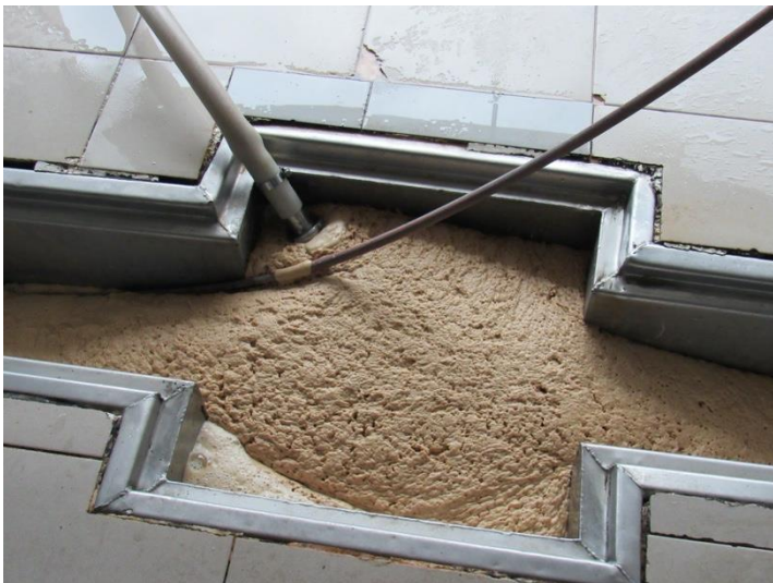
Figure 32: Spent yeast from a fermentation tank being washed down the drain at Birra Stela. Taken on Nov. 12, 2019.
