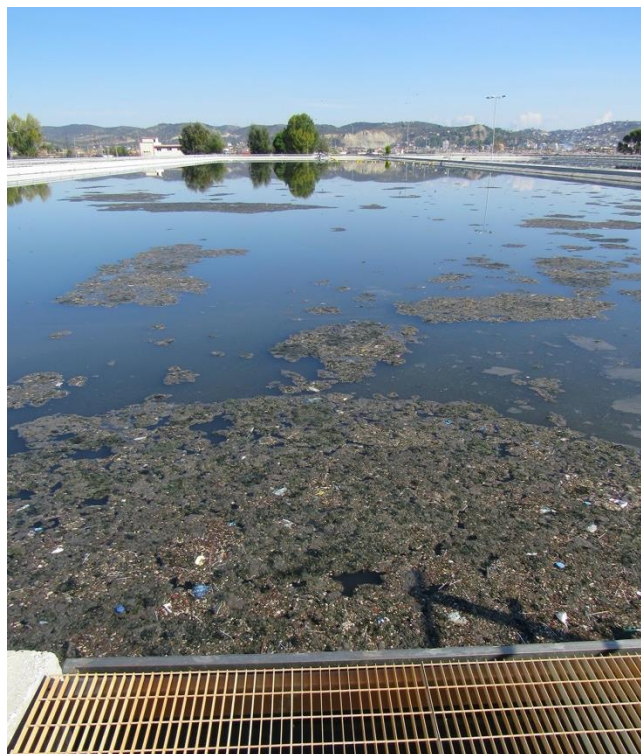
Figure 21: Discharge outlet at Vlorë WWTP. Taken on Nov. 1, 2019.
