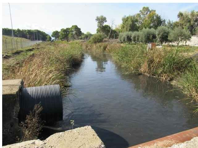
Figure 22: Discharge canal at Vlorë WWTP. Taken on Nov. 1, 2019.
