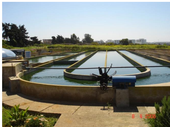
Figure 12: An example of a microalgae treatment raceway pond. This configuration optimizes sunlight exposure (Breedon, 2017).
