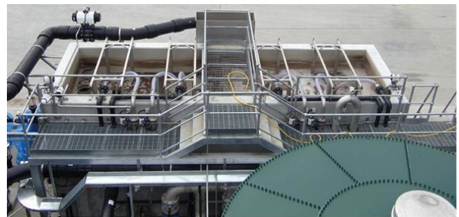
Figure 6: Bluetongue Brewery's aerobic membrane bioreactor post-treatment stage. Water in this stage aerates in a mixing tank to supply oxygen to the microorganisms (CST Wastewater Solutions, n.d.).
