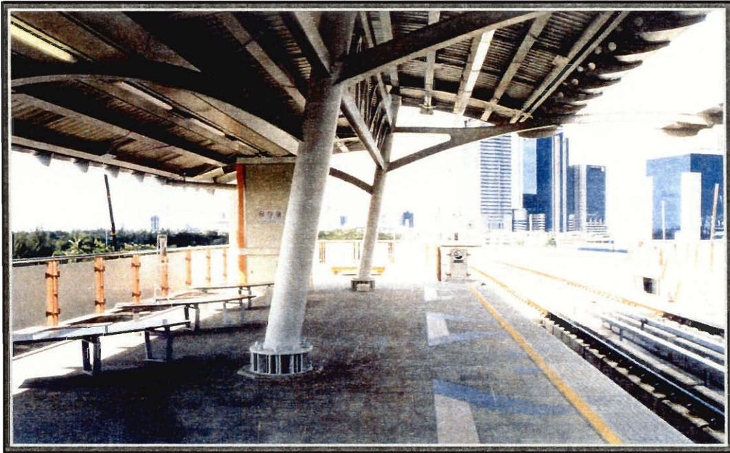
The Central station is of a center platform design with two platforms, one above the other. This permits the direct transfer of passengers between lines. This type of design is a platform located at the center of the station and tracks running along the outer rims. Whilst this layout facilitates passenger transfers from one line to another, construction of stations using this design is more complicated because of the need to curve tracks around the platforms.
