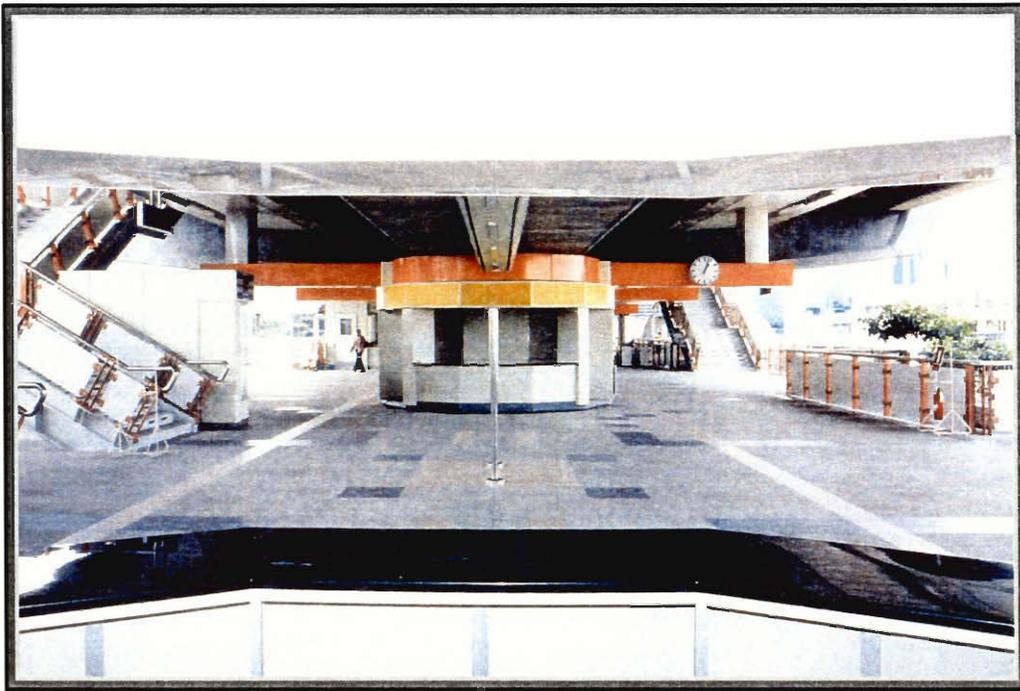
Stations are built on columns erected, where possible, in the central median of the roadways. This type of construction is used so that the maximum road surface is maintained while, at the same time, minimizing diversion of existing utilities necessitated by the construction of the System. Stations are located No. 800 to 1,000 meters apart. Each station is approximately 150 meters long. With the exception of
