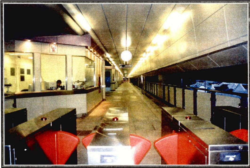
Automatic gates (AGs) are provided on the station concourse level to separate paid and unpaid areas of station. The functions of AGs are to control passengers entering the system and to inspect, update and control passengers' tickets.
