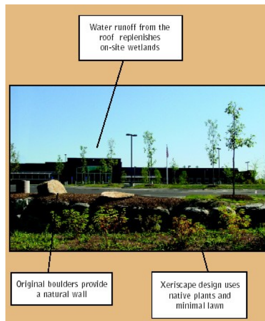
Figure 1: A green building with water efficiency techniques implemented. Xeriscape is an organization that promotes water efficient landscaping. (EPA New England Regional Laboratory Brochure, 2001)
