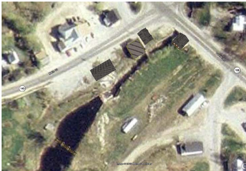
Figure 43: Overview of Site
