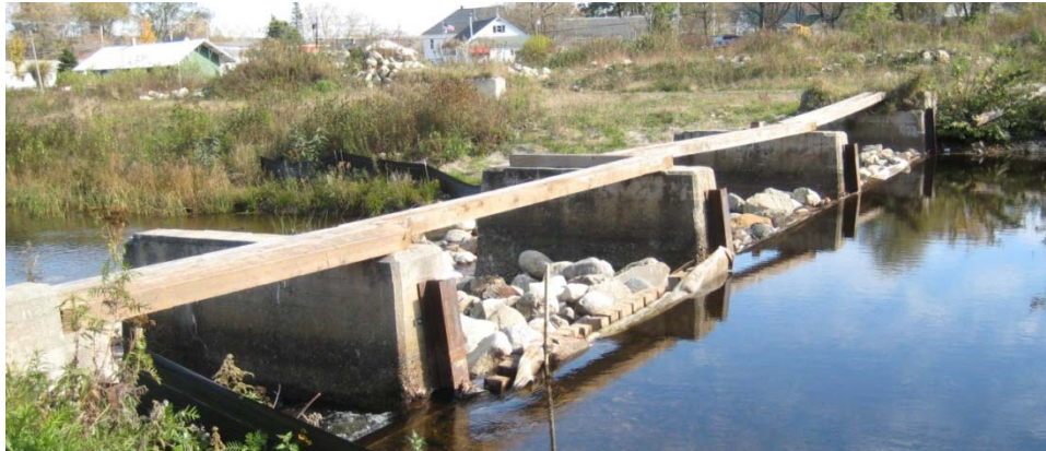
Figure 5: Dam Where Proposed Bridge Will be Located
