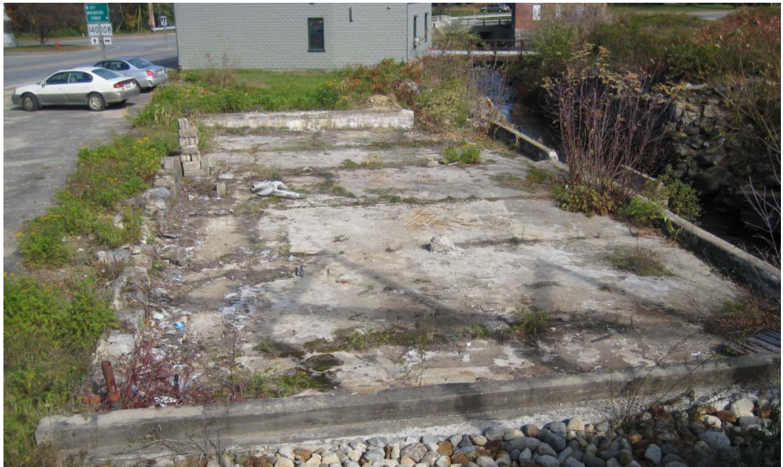
Figure 12: Existing Slab in Lot
