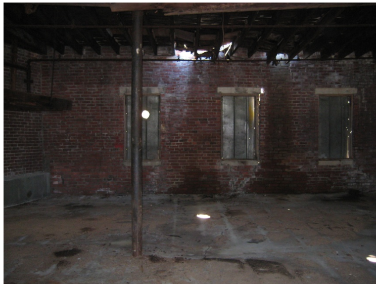
Figure 9: Current Firehouse Interior View
