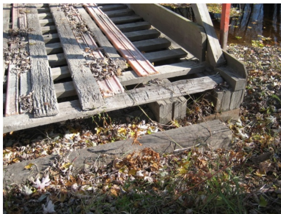
Figure 6: View of Proposed Bridge for Reuse
