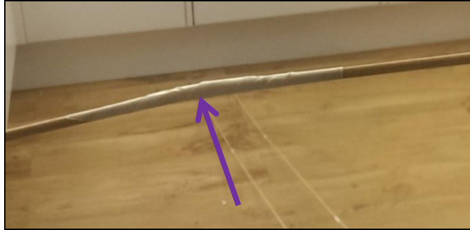
Figure B: The temptation will be to just tape where the joint is, but this won't work well. Apply tape liberally. The arrow shows where the joint is. The taped section here is about 10cm long.
