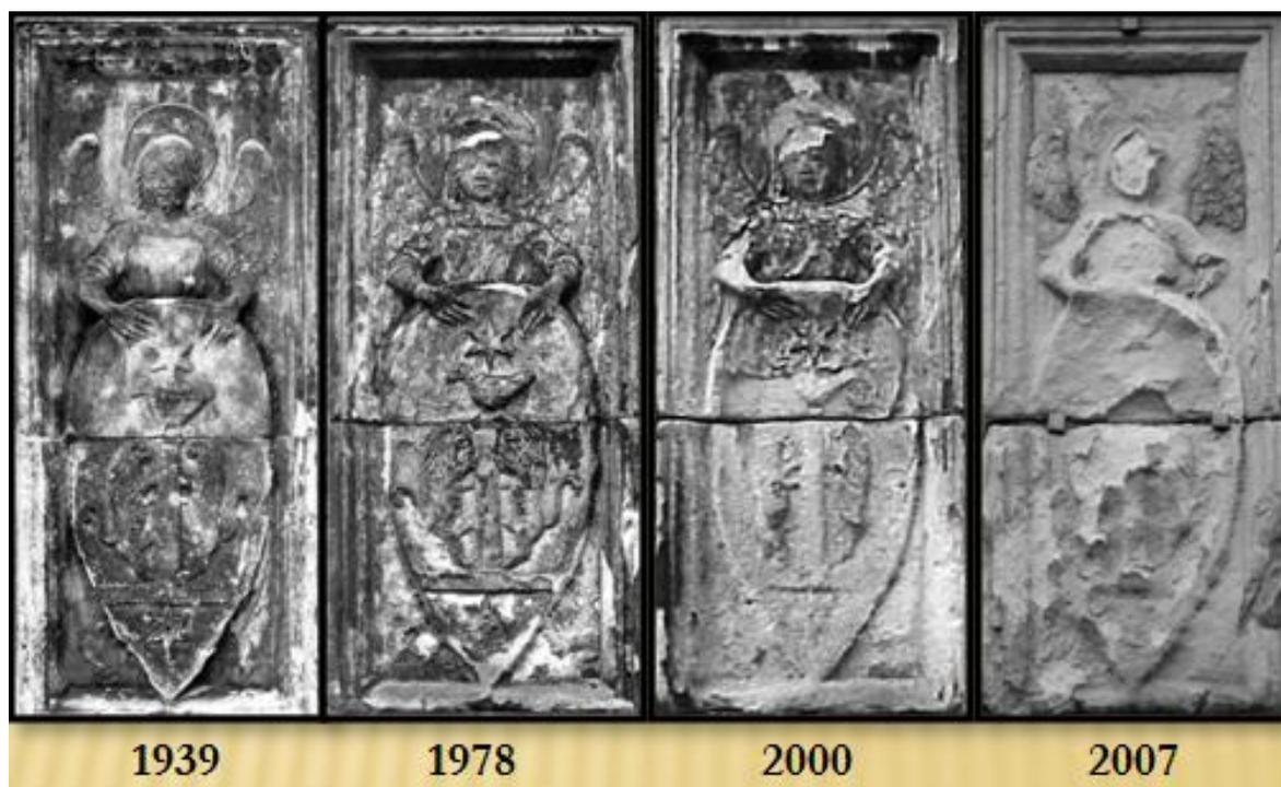
Figure 25 - Angel Deterioration Over the Years
