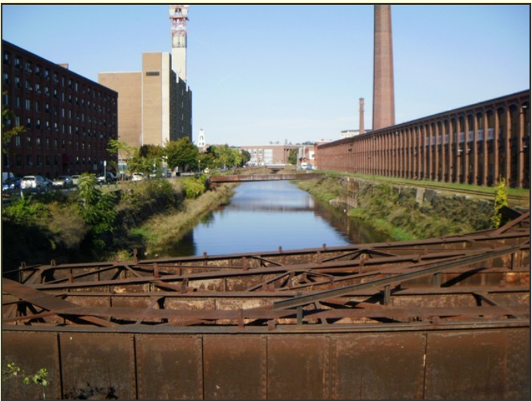
2. Figure 14: Unused Rail Structure over the North Canal
