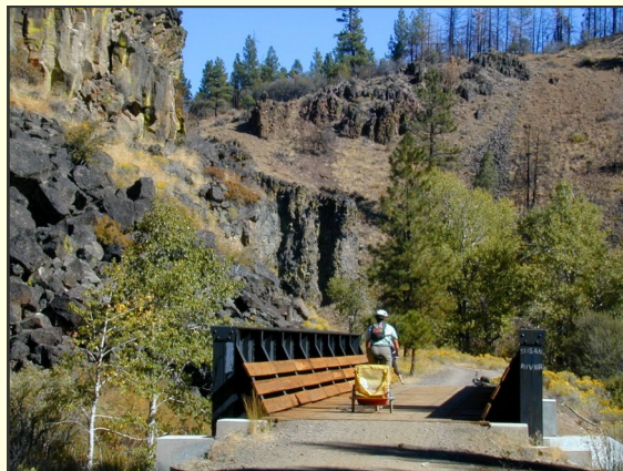
Figure 74: A Bridge along the Bizz Johnson Trail in California 33
