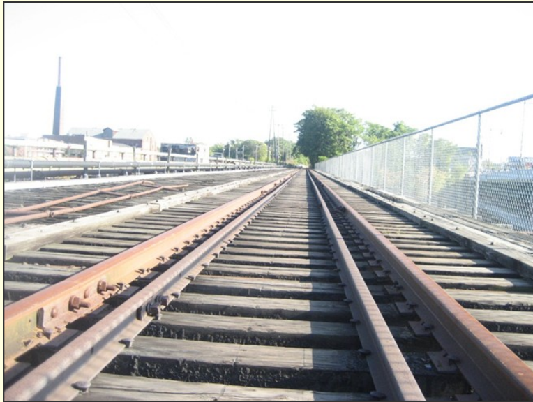
1. Figure 67: Rail Bridge adjacent to the O'Leary Bridge
