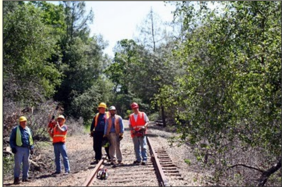
Figure 85: A Contractor along the Danvers Rail Trail are removing overgrown vegetation 37
