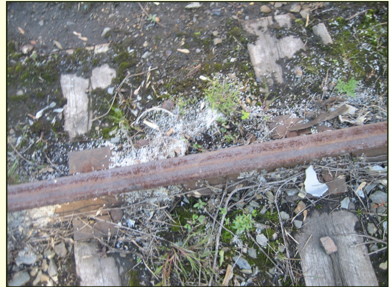
5. Figure 76: Small Plastic pellets scattered along the segment
