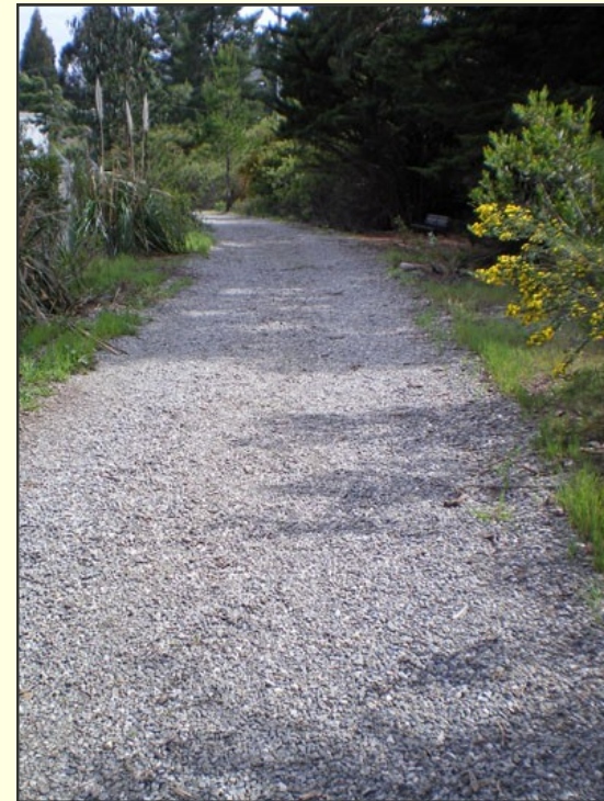
Figure 129: Final product of tie removal 56
