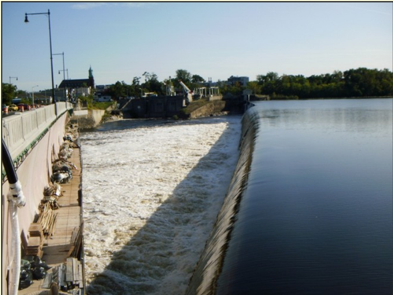
1. Figure 13: O'Leary Bridge and Great Stone Dam
