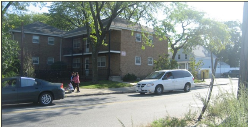
Figure 96: Residential Building on West side of Haverhill Street
