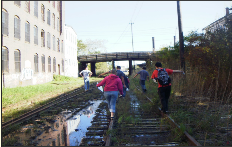
Figure 35: Flooding North of the Lowell Street Bridge
