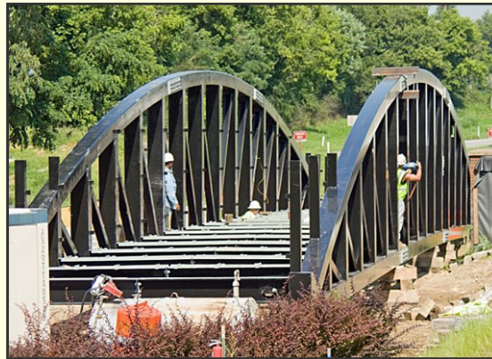
Figure 121: Safety of Bridges include verifying bridge structure 48
