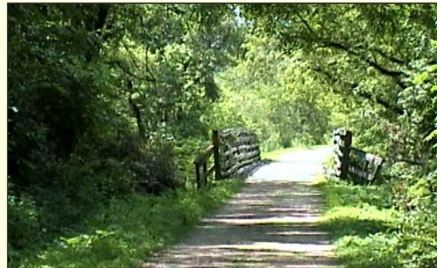
Figure 55: A segment along the Elroy-Sparta bike trail where rustic appeal was maintained 30
