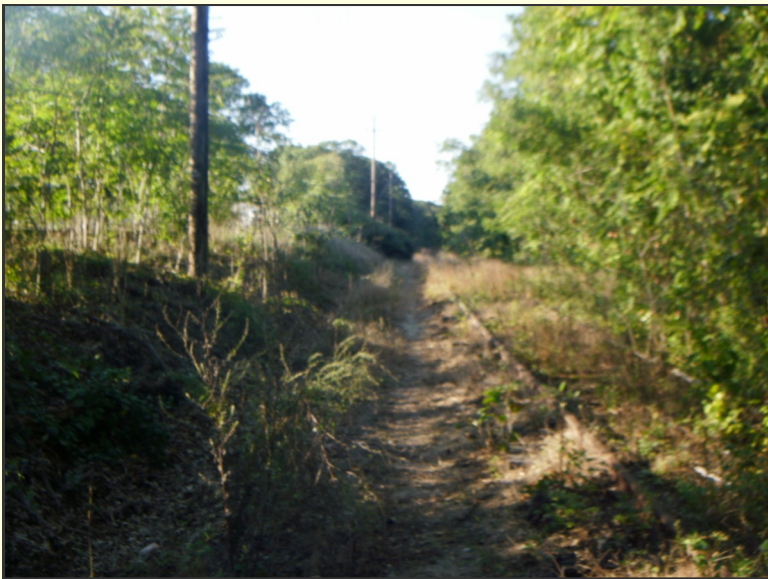
2. Figure 52: The corridor already has a path worn into it
