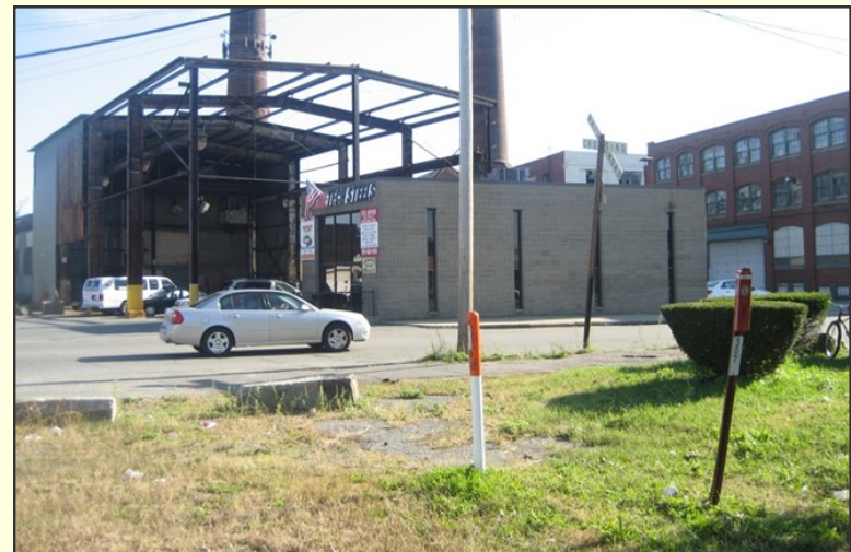
Figure 95: Flame-Tech Steels on Essex Street borders Rail Corridor
