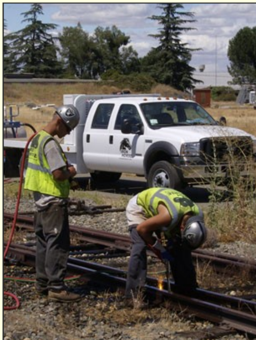
Figure 128: Removal process, Iron Horse Preservation Society 55
