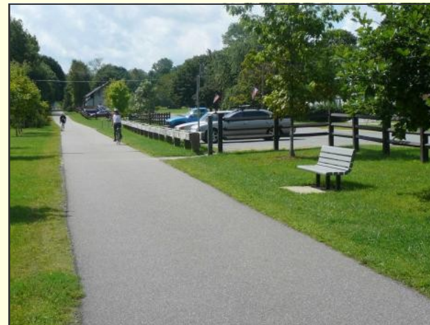
Figure 127: The Ashuwillticook Rail Trail shown includes all the elements of a Rail Trail 54
