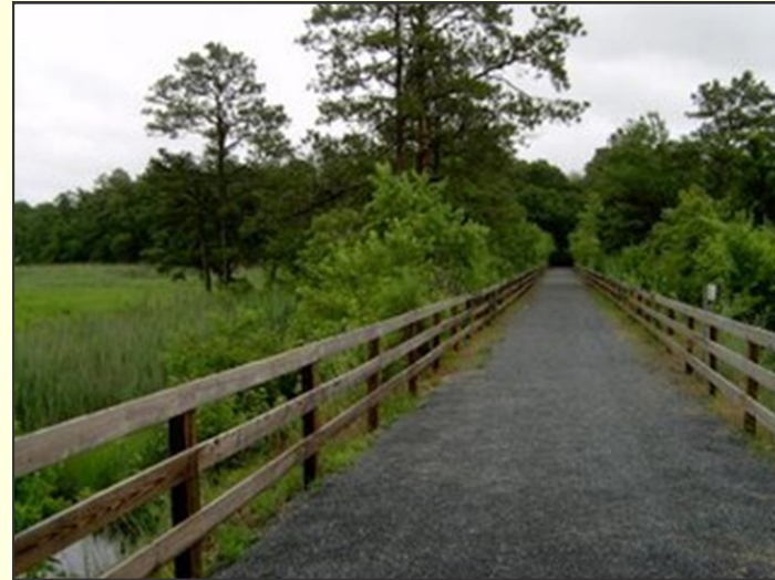
Figure 133: Crushed gravel being used on a current rail trail. 60
