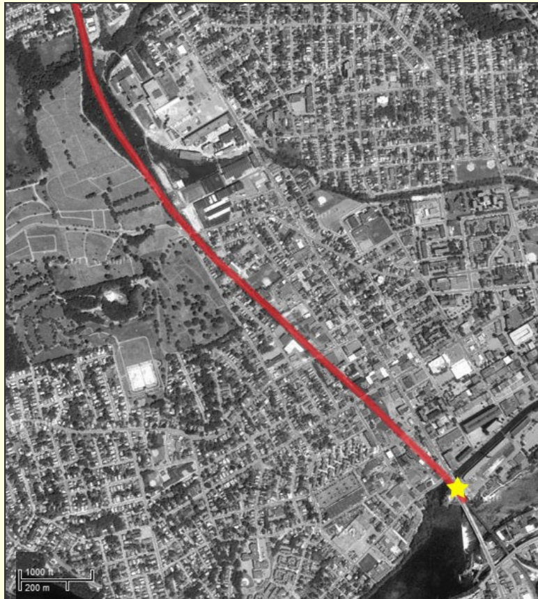
Figure 87: Rail lines cross into the street with no warning
