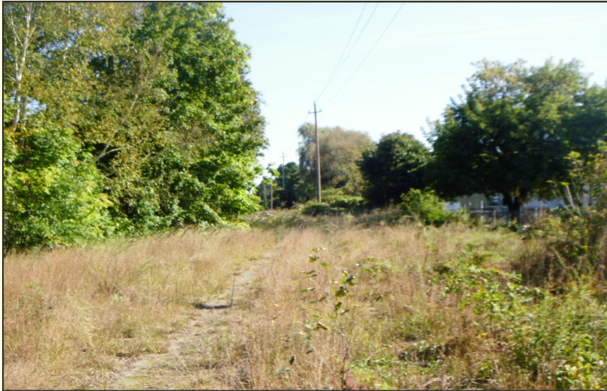
Figure 61: Straight View of Rail Corridor
