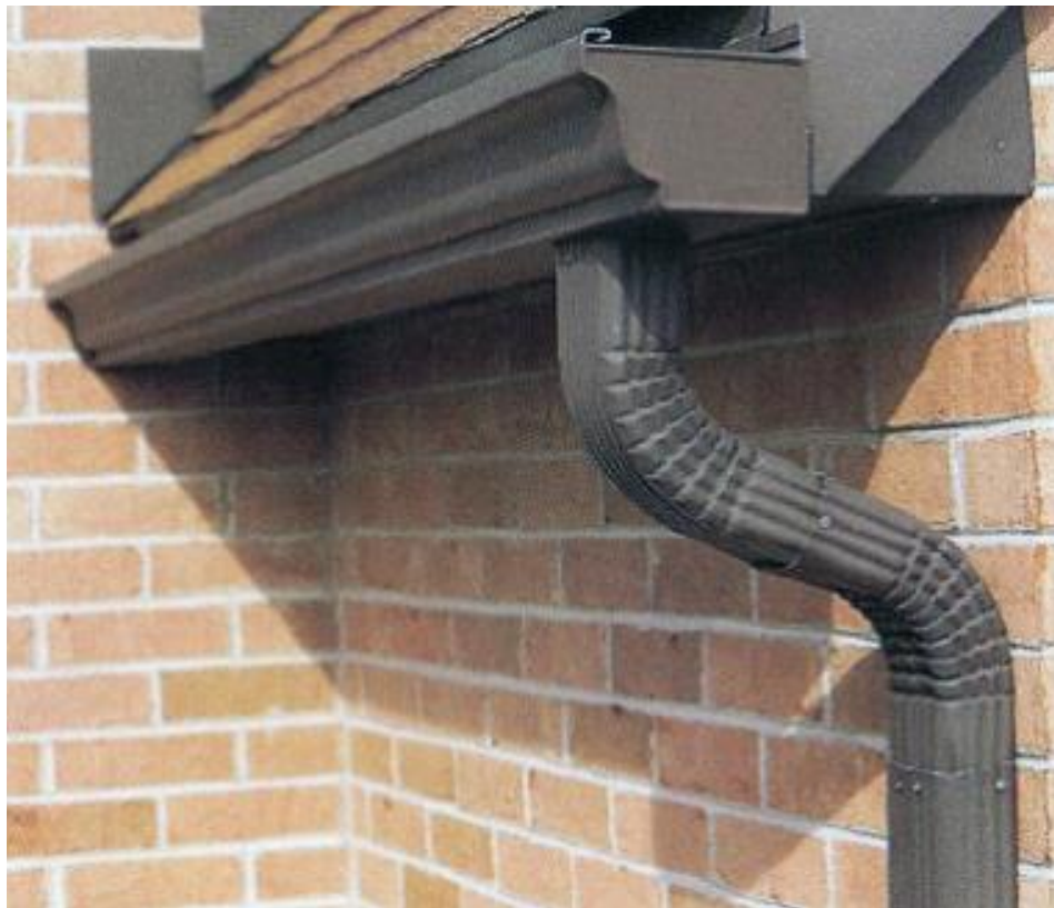
Figure 19: Elbow Connectors and Short Lengths of Downspout
