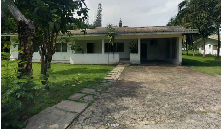
Figure 10: Home in Liberia with Corrugated Roof
