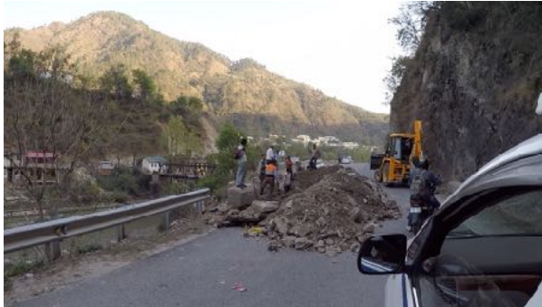
Figure 6: Construction on the road in Kamand on March 27, 2018.
