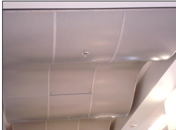
Figure 5: Suspended Ceiling of Hospital de Heredia
