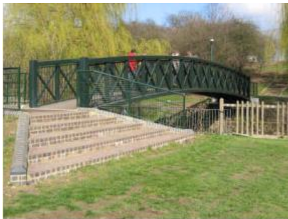
Figure 30. River Brent footbridge (RRC Staff, 2008)
