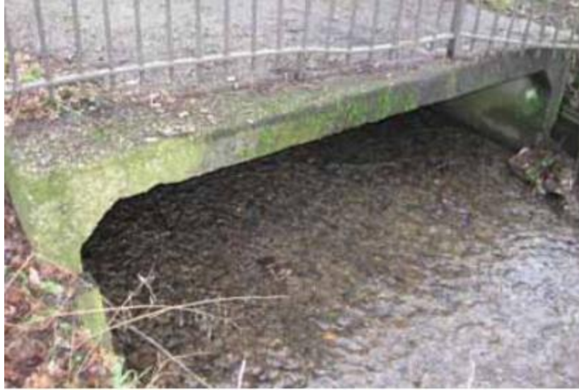
Figure 41. Concrete bridge created during the 1950 channelization (ECRR, 2013)
