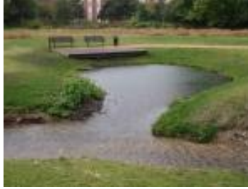
Figure 24. Finished backwater with platform and seating (Case study: Ladywell Fields QUERCUS, 2017)
