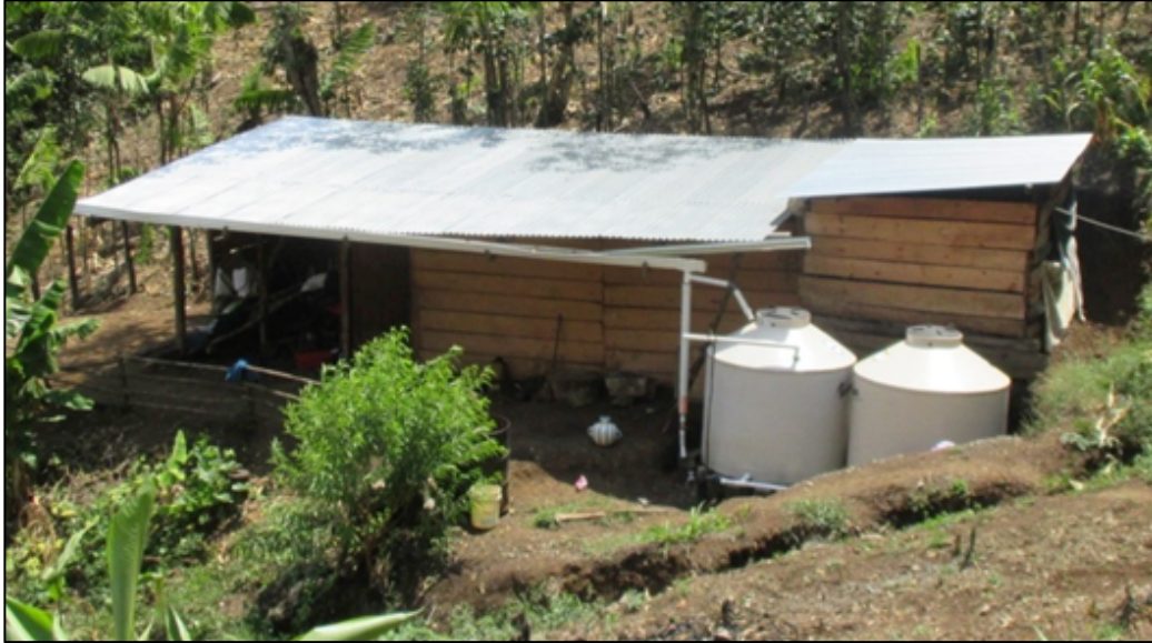
Figure 2: Photo of a corresponding system, built to provide drinking and cooking water to a family in Guatemala. Following three years of research and development, the system featured here was one of 34 constructed by EWB-USA WPI from 2013 – 2015.
