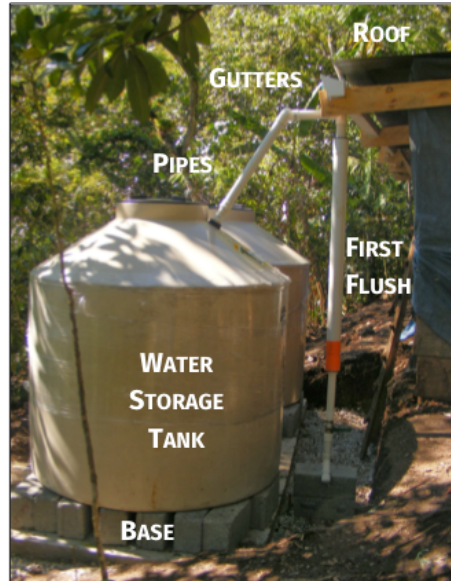
Figure 3: Rainwater harvesting system built by EWB-USA WPI in 2014
