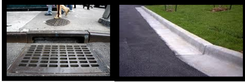
Figure 3: Sewer & Concrete Gutter
