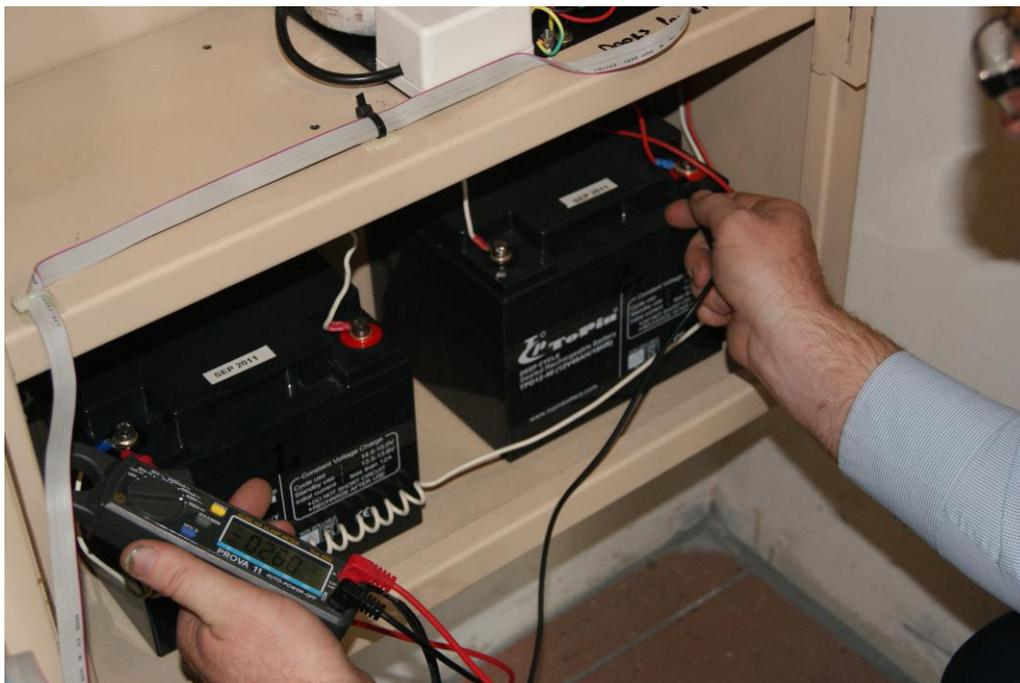
Figure 2: Fire Panel Battery Testing
