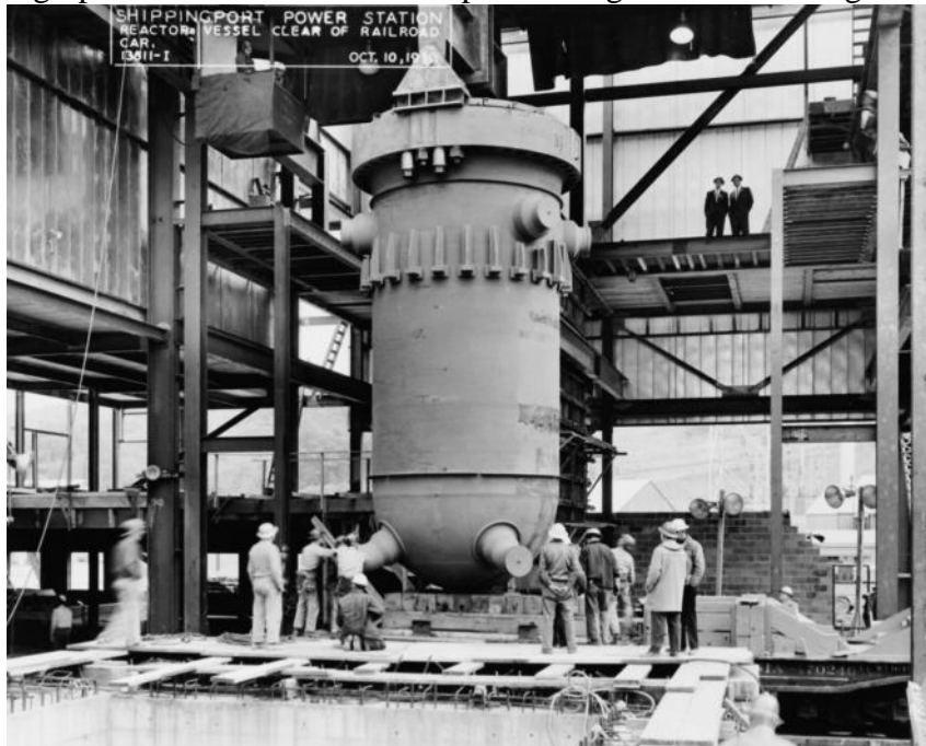
Figure 1: Shippingport Atomic Power during installation; http://en.wikipedia.org/wiki/Shippingport_Atomic_Power_Station
