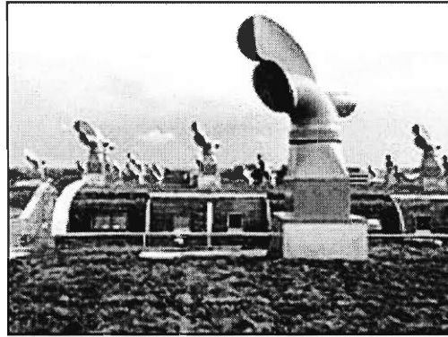
BedZED green roof with wind funnels http://www.greenroofs.com/archives/sq_jan-mar04.htm
