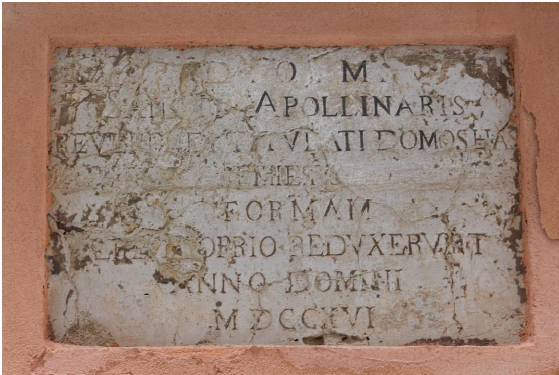
Figure 14 - An Example Inscription With Deterioration
