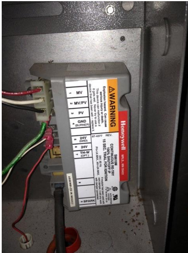
(Figure 19) Ignition Stage Terminals
