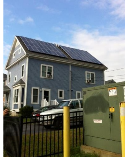
(Figure 5) a residential house with solar panels on the roof, Worcester
