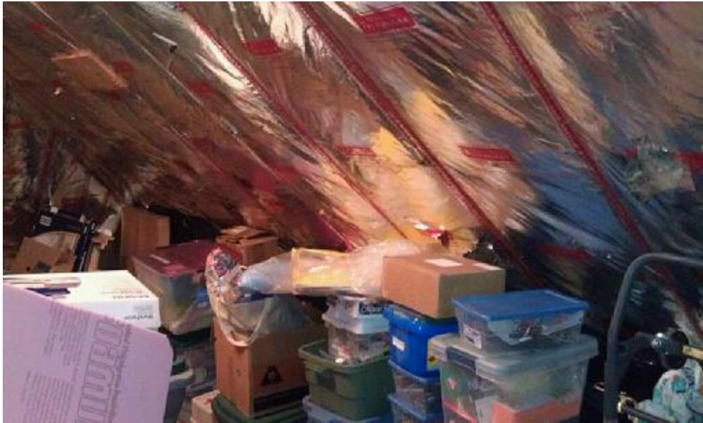
(Figure 14) Current insulation in the meetinghouse attic
