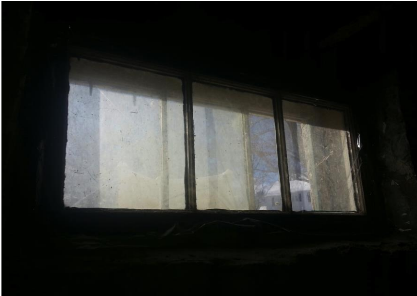
(Figure 22) Window B-11
