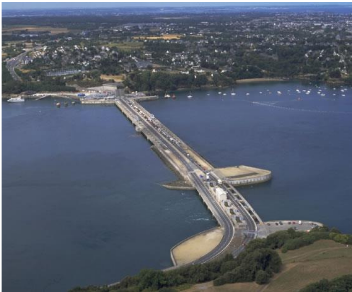
Figure 4-2: La Rance Tidal Barrage [8]
