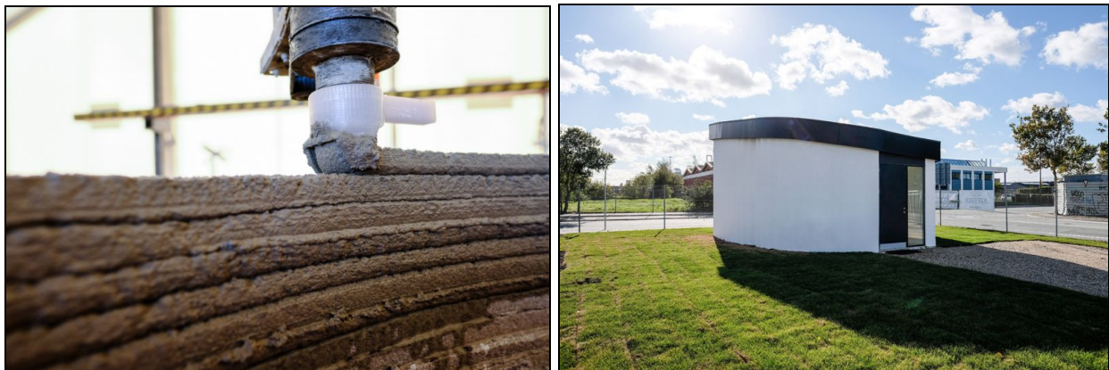
Figure 7: (Left) This image is an up close picture of the COBOD nozzle extruding cement.
