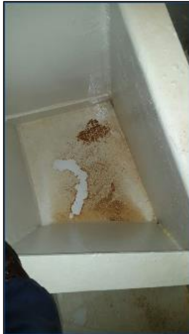
Figure 61: R-GUÍA tank inspection 6-7
