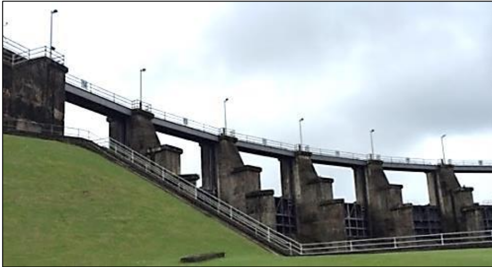
Figure 78: Piers of the Gatun Spillway
