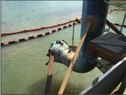
Figure 39: Water Intake at Gamboa
