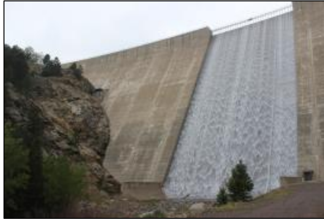
Figure 66: Free falling spillway at Gross Reservoir, CO (Baker, 2013)
