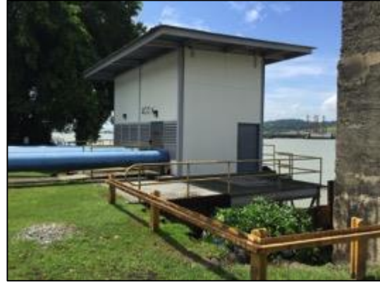
Figure 40: Water Intake at Paraiso
