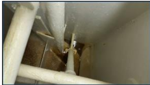
Figure 57: R-GUÍA tank inspection 2-7
