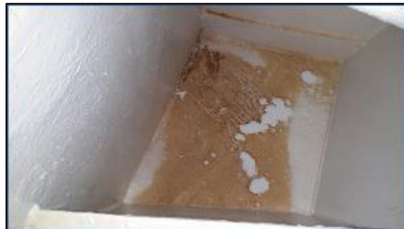
Figure 59: R-GUÍA tank inspection 4-7
