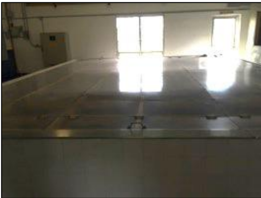
Figure 43: Hydraulic Mixing Chamber
