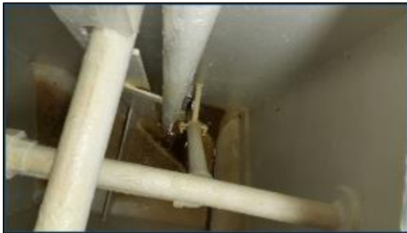
Figure 56: R-GUÍA tank inspection 1-7
