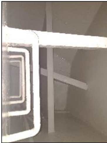
Figure 63: R-GUÍA Potable Water Tank Post Cleaning and Epoxy Painting 1-2
