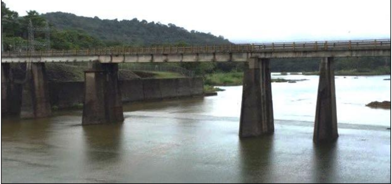
Figure 75: Gatun Spillway traffic bridge
