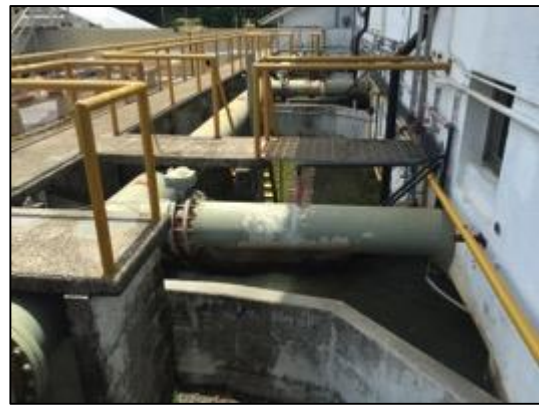
Figure 42: Chemical Batching in Channels
