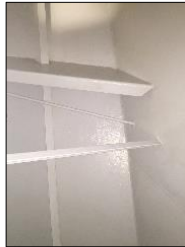
Figure 64: R-GUÍA Potable Water Tank Post Cleaning and Epoxy Painting 2-2
