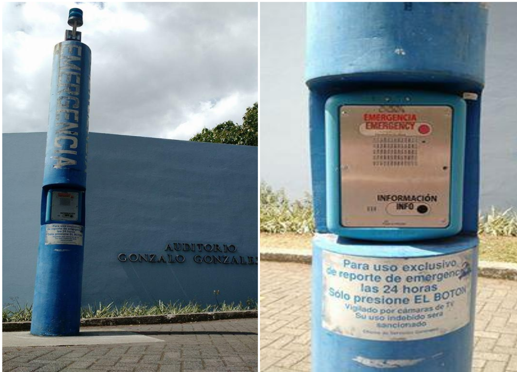
Figure 4.8 This figure shows one of the blue light call boxes and its use description on UCR’s campus.
