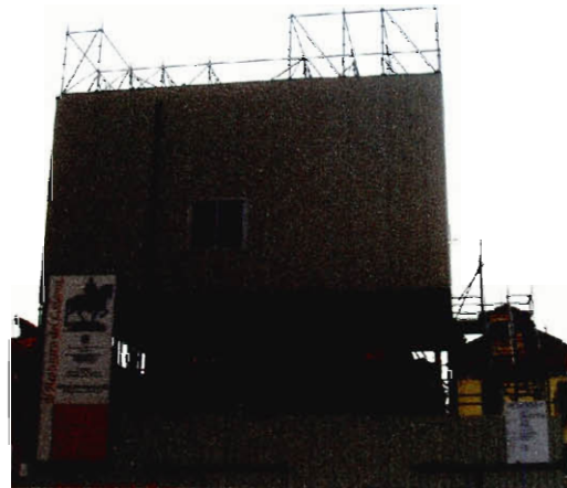
Figure 28: Example of Restoration in Progress
