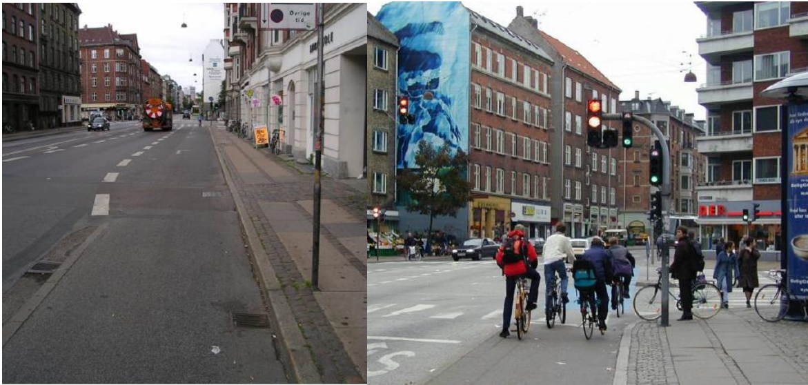
Figure 4: Photos of shortened bicycle track (left) and advanced bicycle track (right) (Jensen, 2007).
