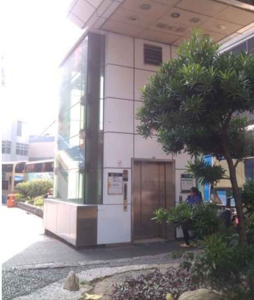
Figure G. 13: Route 8, lift for handicapped access, hidden under the stairs
