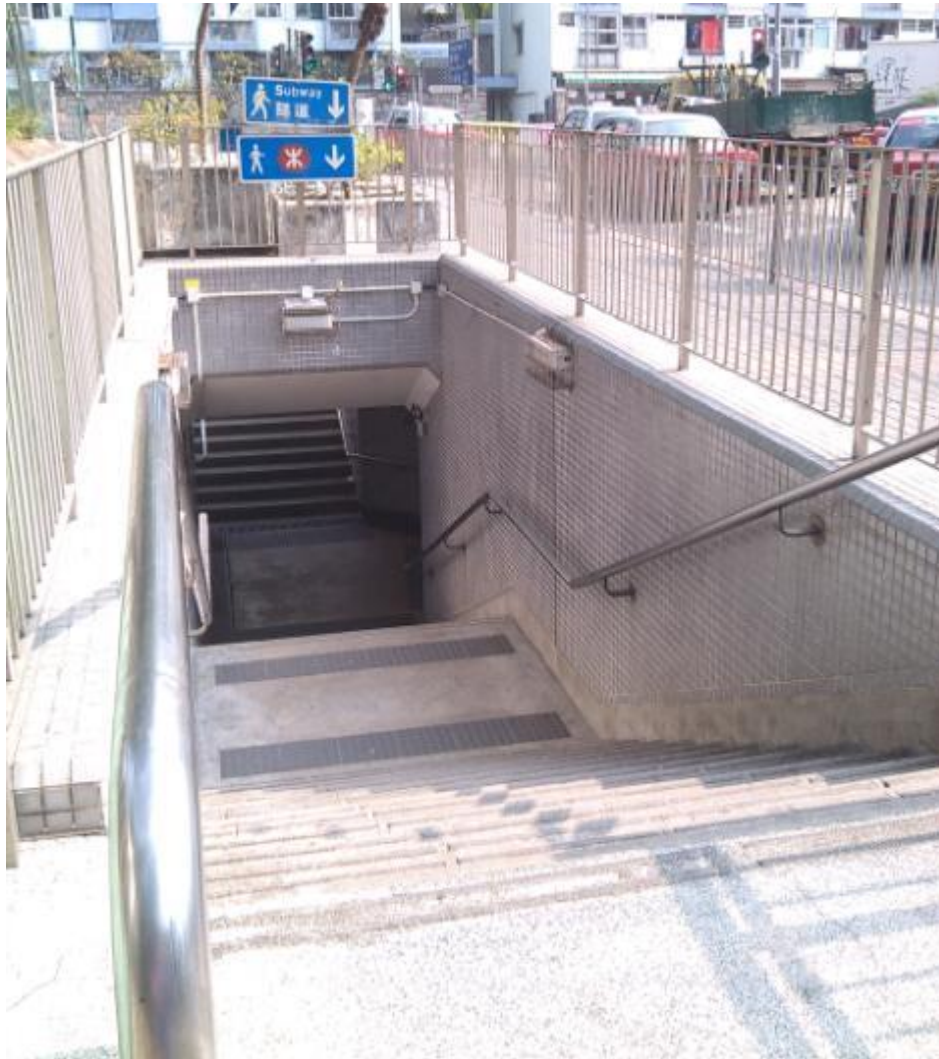
Figure G. 4: Route 3, steps leading to the subway
