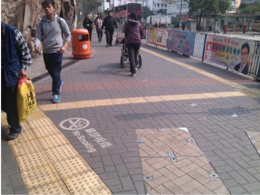
Figure G. 16: Route 10, only tactile surfaces found on sidewalks along Kwun Tong Road
