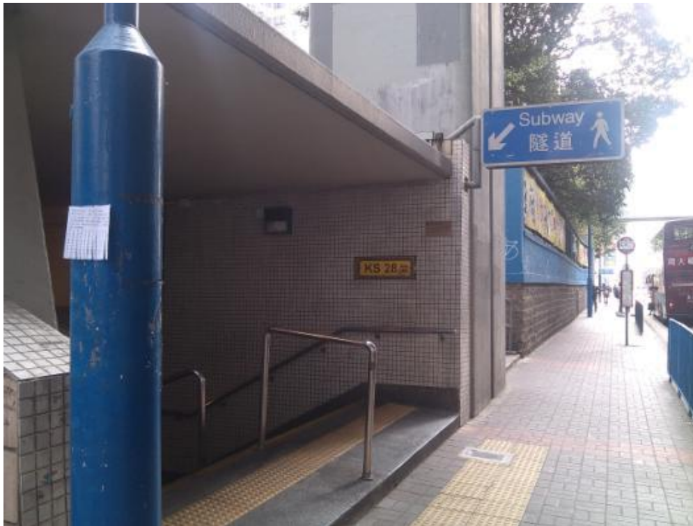
Figure G. 6: Route 5, north entrance on residential side of Kwun Tong Road
