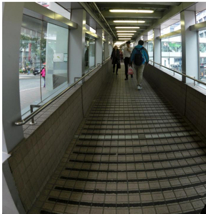
Figure I. 1: Pedestrian Footbridge Ramp
