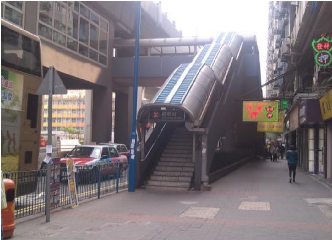
Figure G. 15: Route 10, a pedestrian footbridge that goes to the Kwun Tong MTR Station
