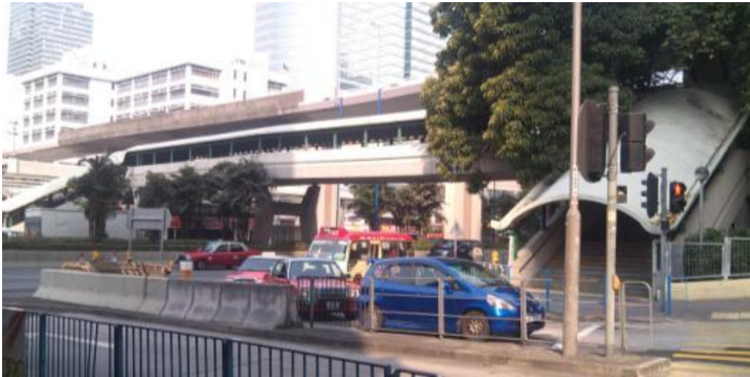
Figure 4.11: Route 1, A Challenging Pedestrian Overpass
