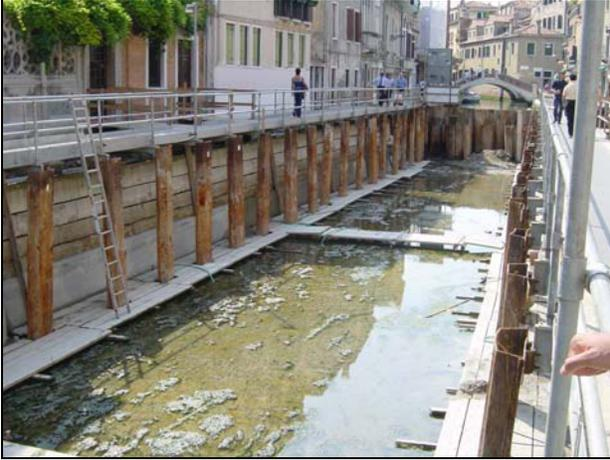
Figure 2-20 A canal undergoing wall repairs
