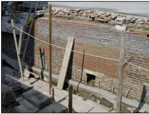
Figure 2-12 Canal Wall Construction: Type of Wall Lining for Fondamente
