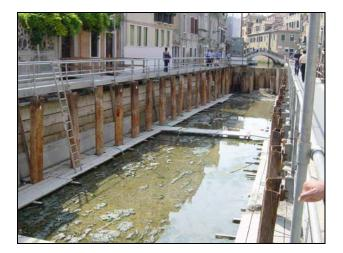
Figure 2-20 A canal undergoing wall repairs
