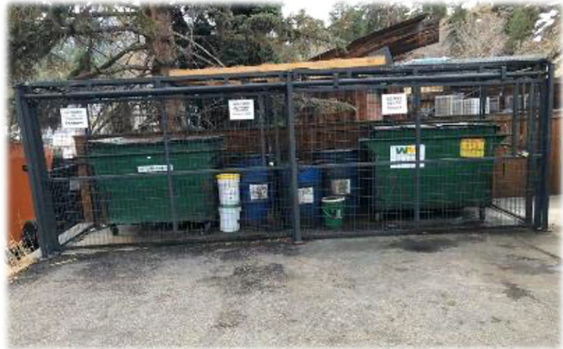
Figure 21. In this picture, cooking oil containers and trash dumpsters are locked inside a large enclosure. This is an effective way to prevent bears from being able to reach the containers at all. The cage is both locked and enclosed on all sides.
