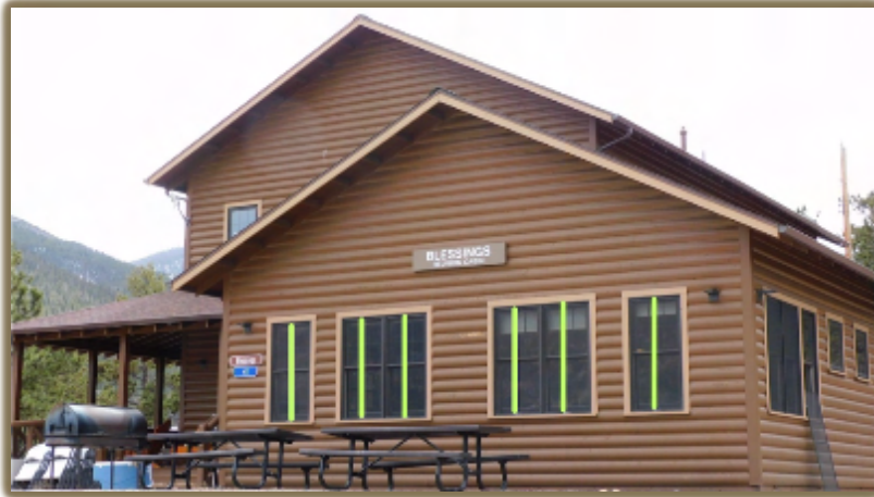
Figure 26. The bars in light green indicate suggestions where metal bars can be placed of the same color and material as the existing window.
