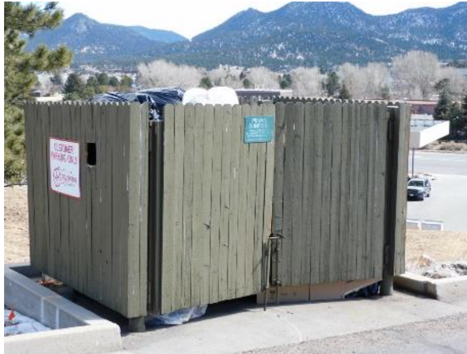
Figure 27. Image of a trash disposal area behind a local business.
