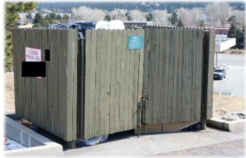
Figure 20. This is an example of a dumpster and enclosure being used incorrectly. The dumpster is overflowing in the top and the fence enclosure would not be effective at keeping bears out since there is no top to it.
