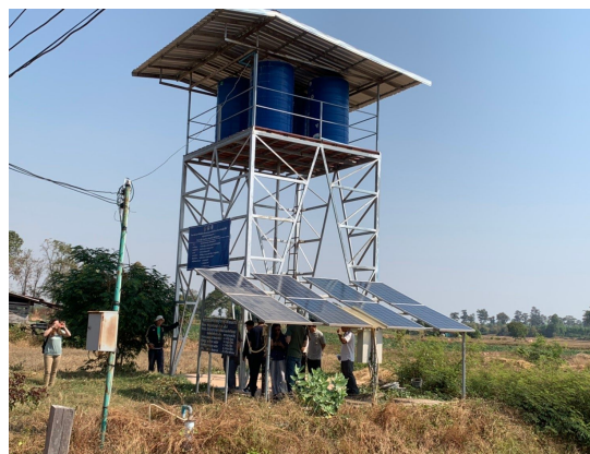
Figure 15. The solar panel and water tank that were installed in Ban Lan
