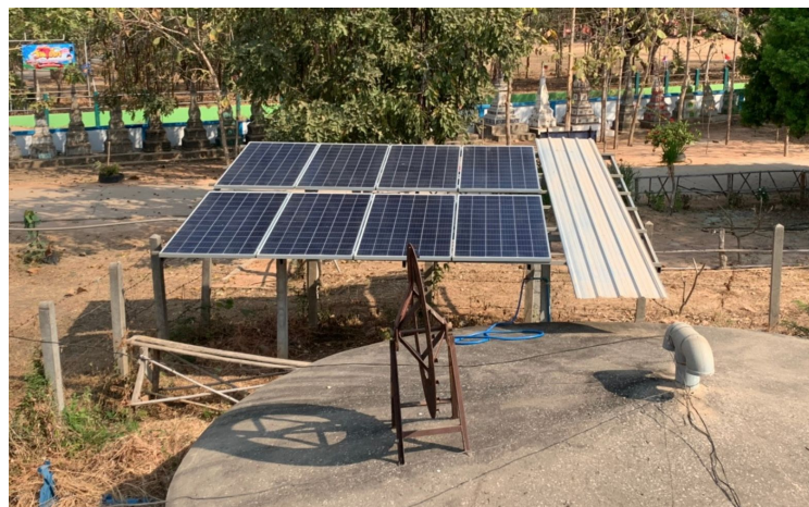
Figure 3: Tilt of a fixed solar array
