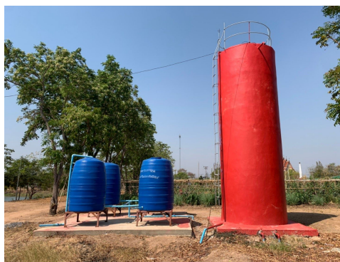
Figure 10: Old tanks (blue) and tank installed by PDA (red)
