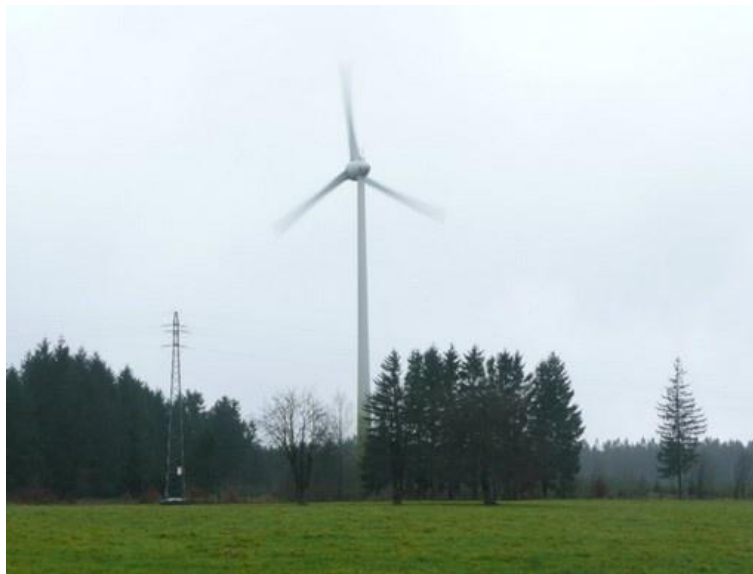
Figure 15: Enercon E33 in Use
