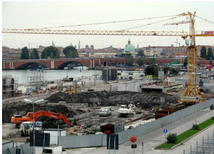
Figure 41: Construction site of the new warehouse in Tronchetto
