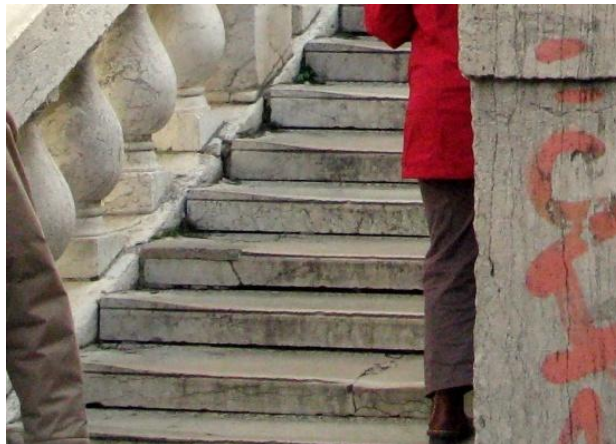
Figure 12: Side stairs on the Rialto worn down due to the passage of tourists
