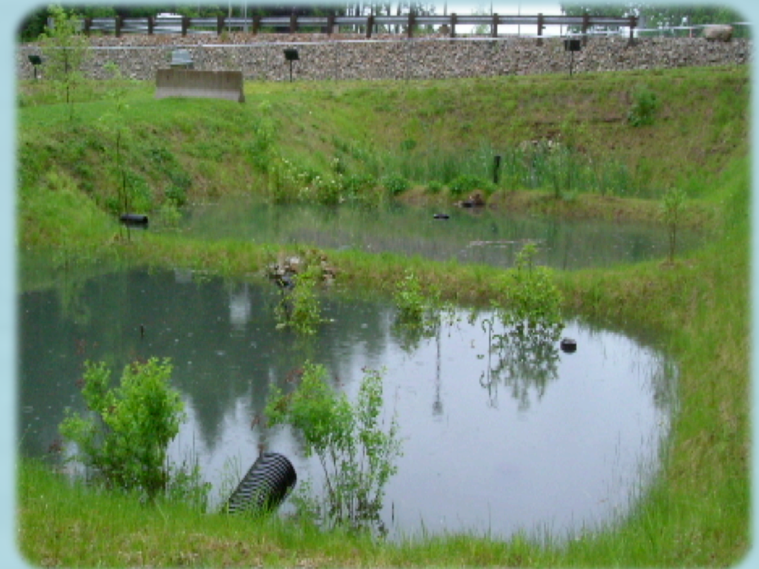
An example of a vegetated basin for water treatment (University of NH. 2009)
