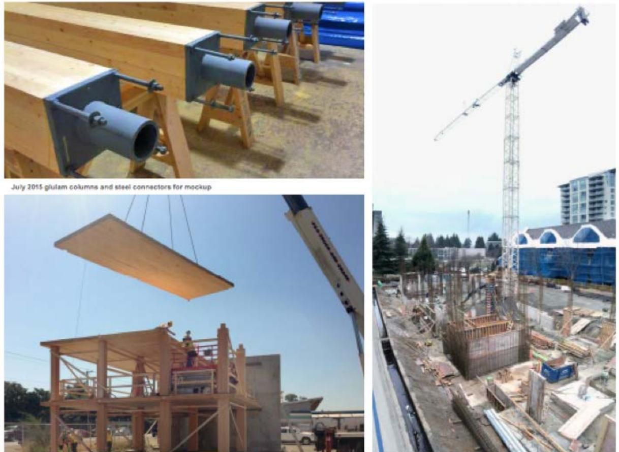
*Figure 3: Mass Timber Construction*
