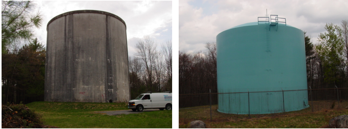
Figure 7: Cement (L) and Steel (R) Storage Tanks
