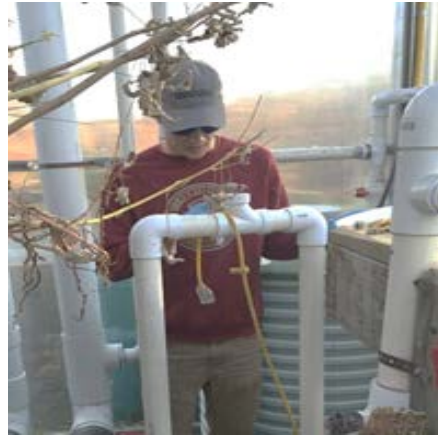
Figure 10: System Effluent Sampling Location
