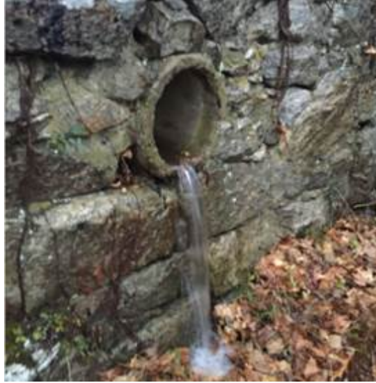
Figure 11: Stormwater- Drainage Pipe Sampling Location
