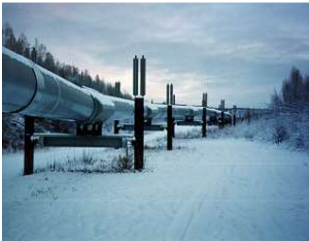
Figure 9.6: Longest oil pipeline on Earth as comparison
